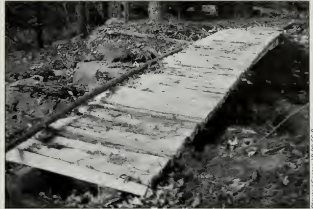
Fig. 5-25 This corduroy bridge was constructed in 1998 by the Northeast Harbor VIS below Asticou Gardens on the Asticou Brook Trail (#514). Rough split cedar decking is laid on stripped cedar log stringers and supported by stone abutments.
