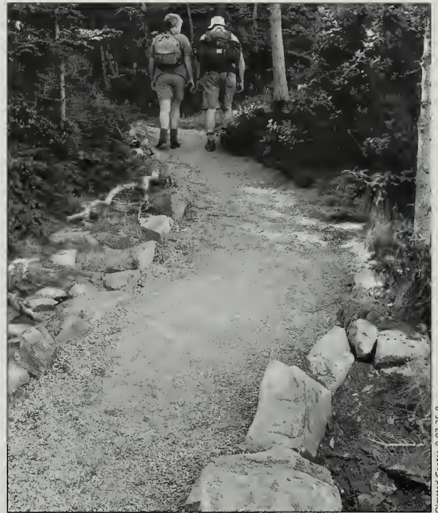
Fig. 6-8 Rehabilitated section of the Ocean Path (#3) with new tread.
