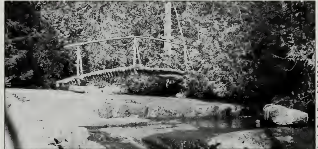
Fig. 5-26 This arched corduroy bridge with a single railing was constructed by the Northeast Harbor VIS circa 1998 on the Lower Hadlock Trail (#502). The cedar stringers are naturally curved logs, typical of trees found along pond shores or stream banks.
