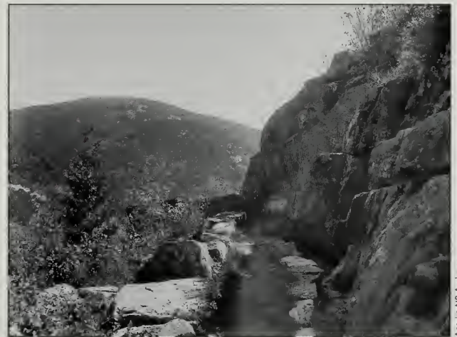
Fig. 4-10 A 1920 view of capstone culvert with walled side drain on the Emery Path (#15) constructed in 1916 by Bar Harbor VIA.
