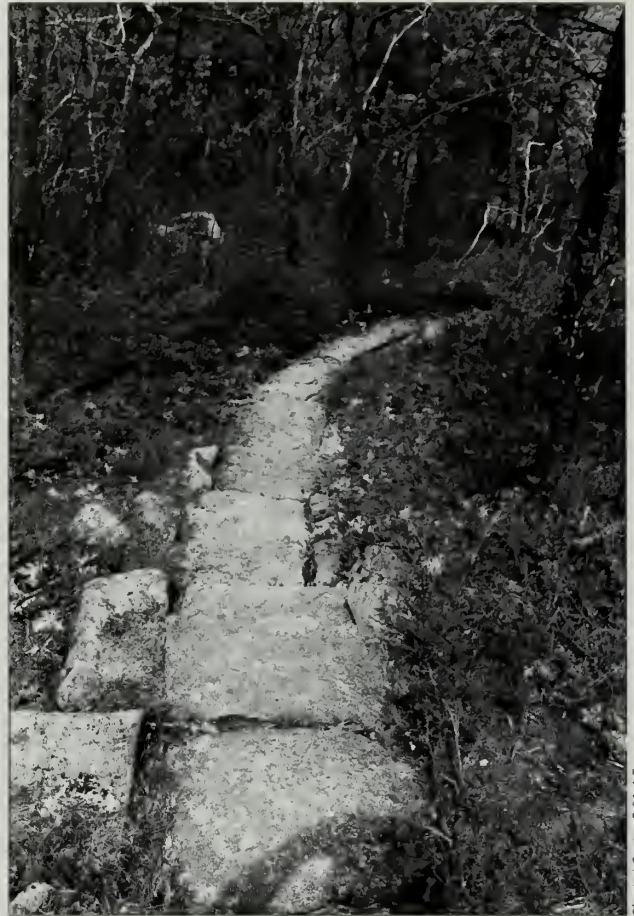
Fig. 15-10 Stone paved trail and steps in good condition.
