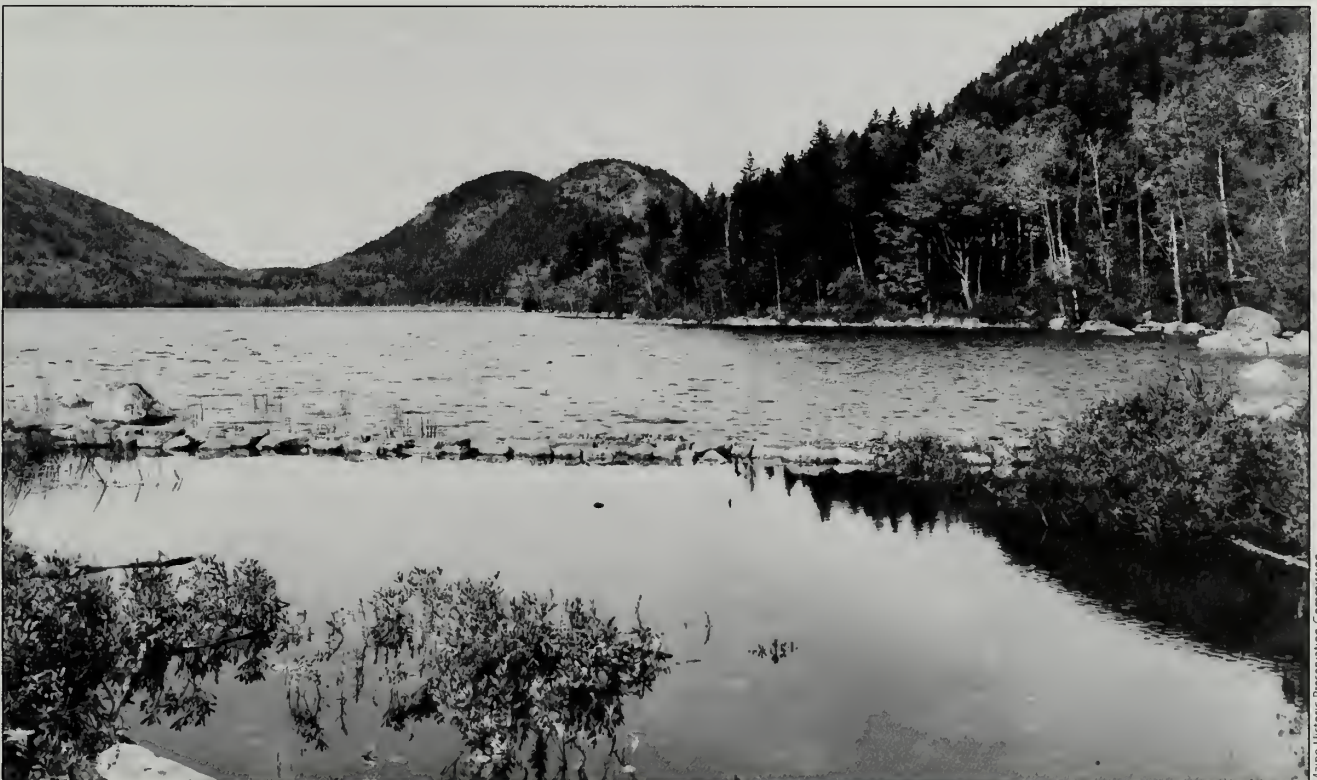
Fig. 3-19 An early photograph of the Jordan Pond stone causeway, circa 1920. Note the small rocks, narrowness, and unevenness of the causeway, which would not well accommodate today's number of users.
