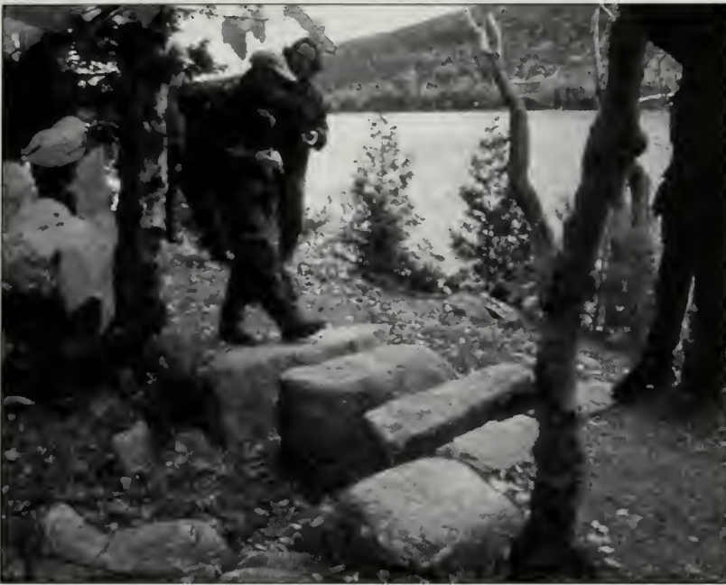
Fig. 4-27 Newly installed stepstone culvert on the Jordan Pond Path (#39).
