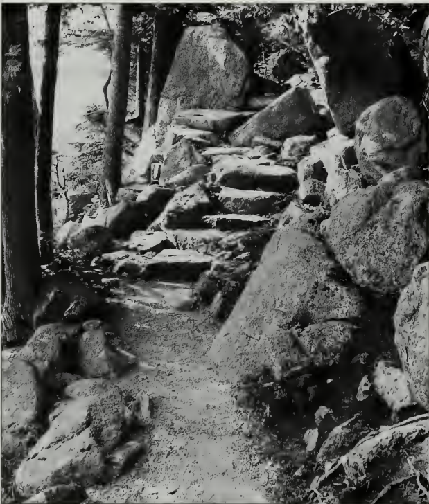
Fig. 7-43 NPS rehabilitation of Bates-style steps on the same section of the Jordan Pond Path (#39) in 2002. Note varying sizes, flat "patio" above the fifth step, and use of both slab-laid (top step) and set-behind (front steps). Steps also conform to boulders in the landscape.
