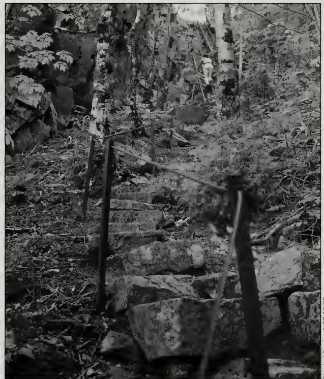
Fig. 8-31 Cable on stanchions on the Beech Cliff Ladder Trail (#106).
