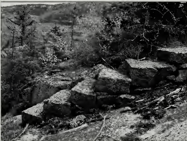
Fig. 349-23 Stone steps pinned on ledge, side view.
