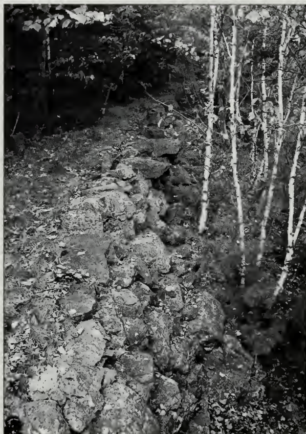
Fig. 6-25 An original rubble-laid retaining wall on the abandoned Gurnee Path (#352).
