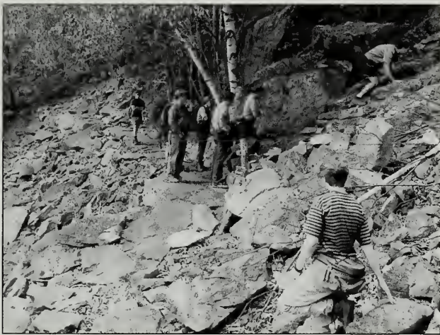
Fig. 3-32 Talus pavement on the Champlain East Face Trail (#12).
