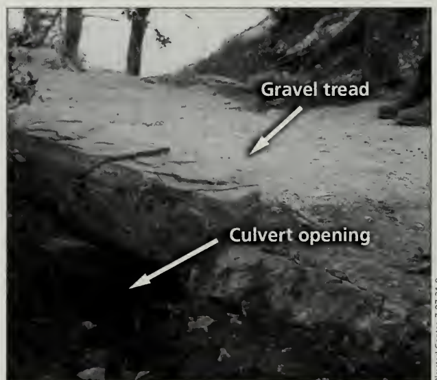
Fig. 4-3 A graveled-over culvert on the Ocean Path (#3).
