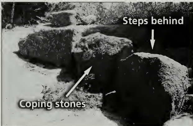
Fig. 7-19 The stone steps on the Van Santvoord Trail (#450) were often located on ledgerrock where there is no apparent need for a set of steps. These steps functioned more as a route guide than an aid to traversing the slope.
