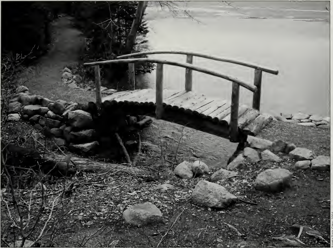
Fig. 39-1 Corduroy bridge built in 2004 on the Jordan Pond Path near the Jordan Pond Carry Path.
