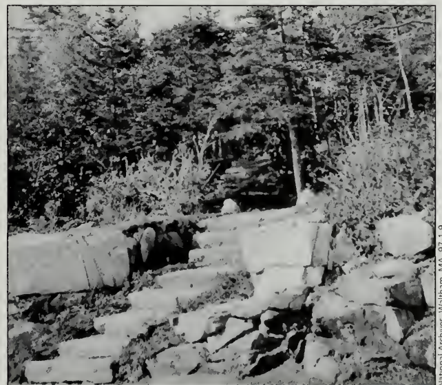
Fig. 7-29 CCC steps connecting Ocean Path (#3) with a parking area along Ocean Drive, soon after construction, circa 1937.
