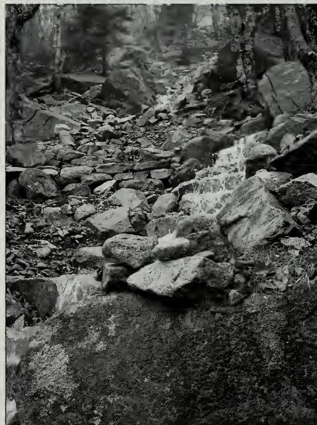
Fig. 48-16 Tread and slope stabilization in progress in 2004 using winding steps built in the VIA/VIS style.
