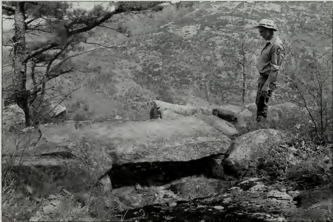
Fig. 15-11 Massive capstone culvert.
