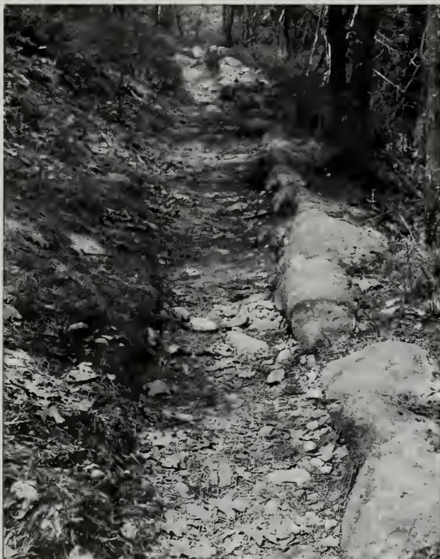
Fig. 15-14 Low coping wall holding water on tread.
