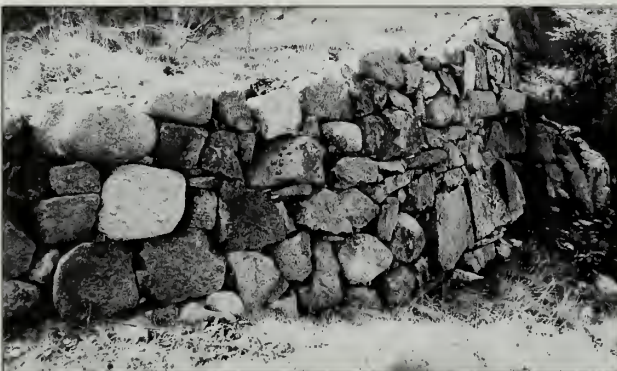
Fig. 6-42 This rehabilitated laid stone retaining wall on a section of the Ocean Path (#3) was completed by the Acadia trails crew in 2000.
