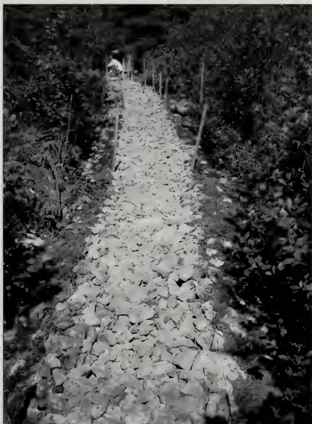
Fig. 3-26 Wall-less causeway before gravel surfacing on the Jordan Pond Path (#39) in 2002. The sides are angled and revegetated to the grade line. Note the insloping culvert lintels between first and second grade stakes.
