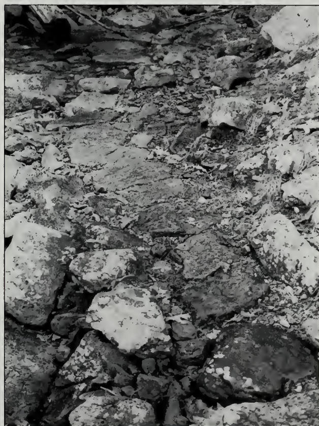
Fig. 3-34 VIA tread pavement on the Gorge Path (#28).
