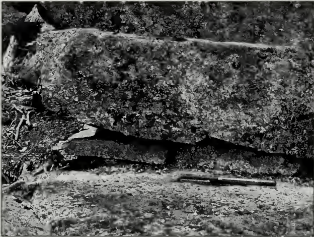
Fig. 349-21 Stone step with shims.
