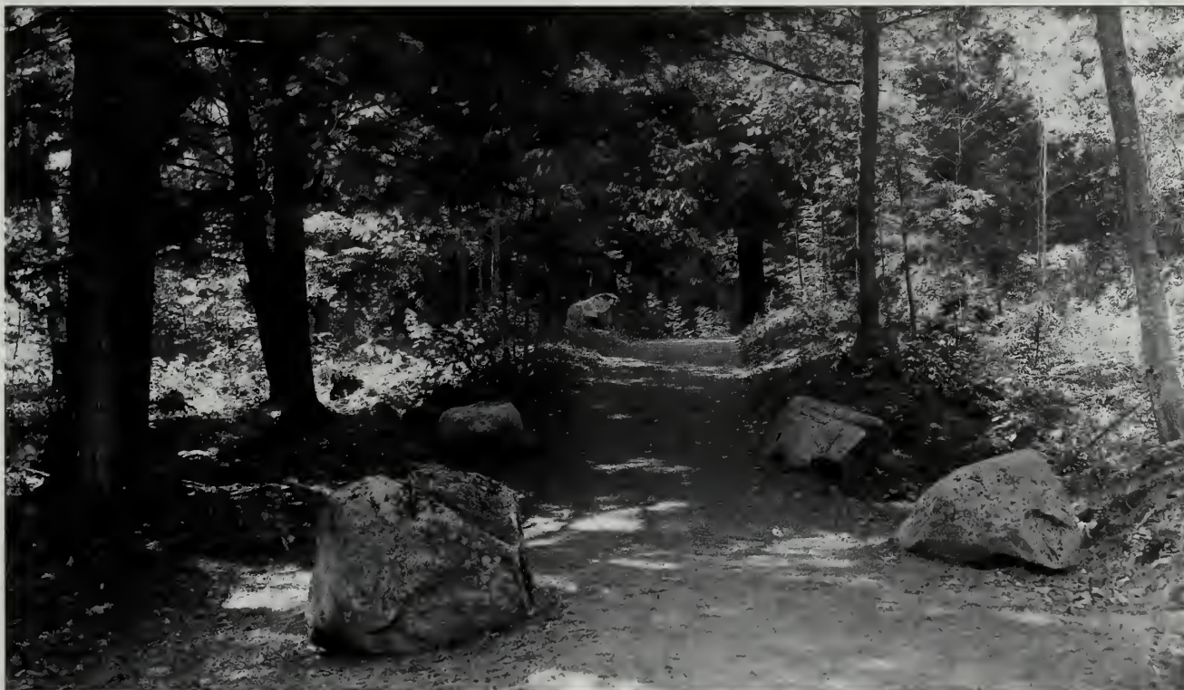
Fig. 6-11 Large and medium-sized coping stones defining the edges of the Stratheden Path (#24), circa 1920s.
