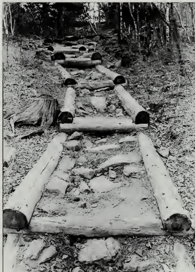
Fig. 6-54 Treadway cribs on the Bear Brook Trail (#10).
