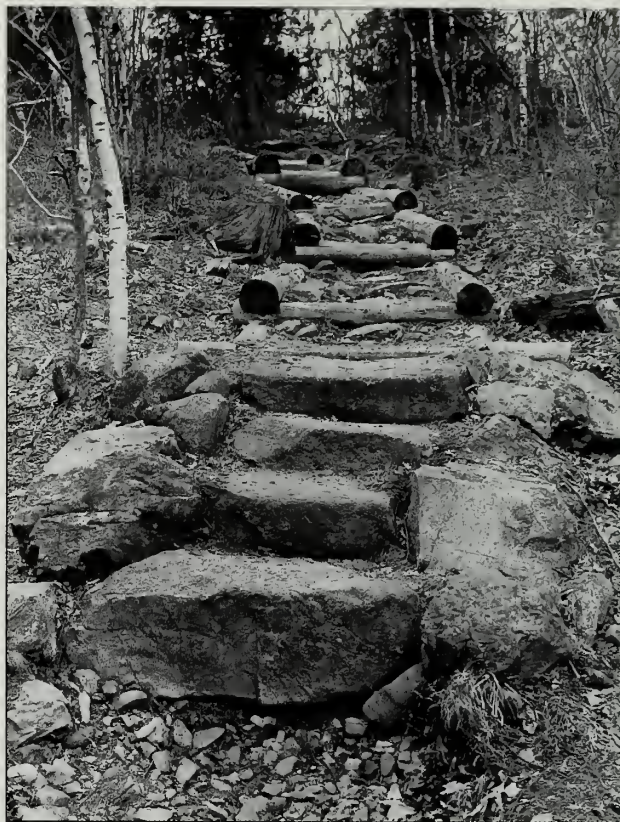
Fig. 1-5 The Bear Brook Trail (#10) was an early route later stabilized with trail features like these stone and wooden crib steps.
