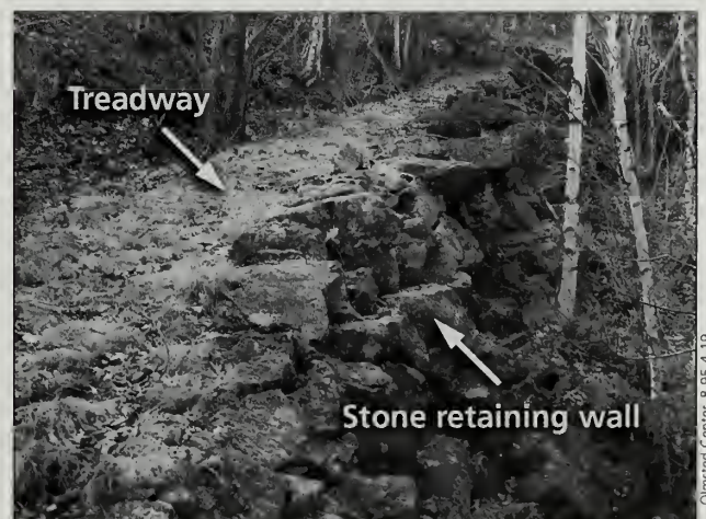
Fig. 3-3 This bench cut on the Gurnee Path (#352) is supported by stone retaining walls on the downslope side.
