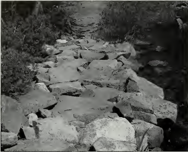
Fig. 3-24 This stone causeway on the Great/Long Pond Trail (#118) was constructed in 1993 by the NPS; however, it is out of character for this trail and should be replaced with walled or wall-less causeway.
