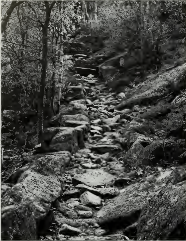
Fig. 15-5 Gravel surface has washed away, exposing rubble base.
