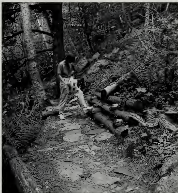
Fig. 6-53 A wall crib on the Beech Cliff Ladder Trail (#106).
