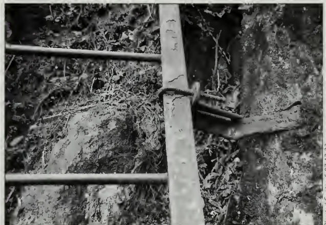
Fig. 8-32 Fastener for ladder on the Beech Cliff Ladder Trail (#106).
