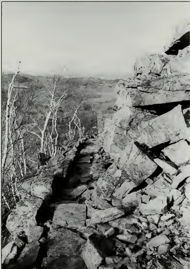
Fig. 6-17 Evenly spaced coping stones on the Beachcroft Path (#13).
