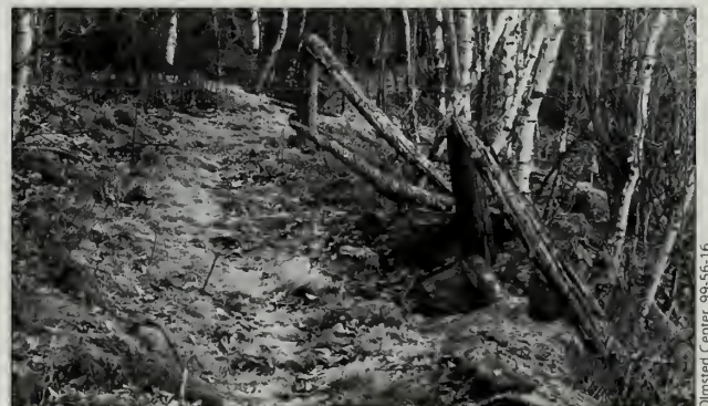
Fig. 9-56 Extant VIA/VIS railings on the abandoned Gurnee Path (#352).
