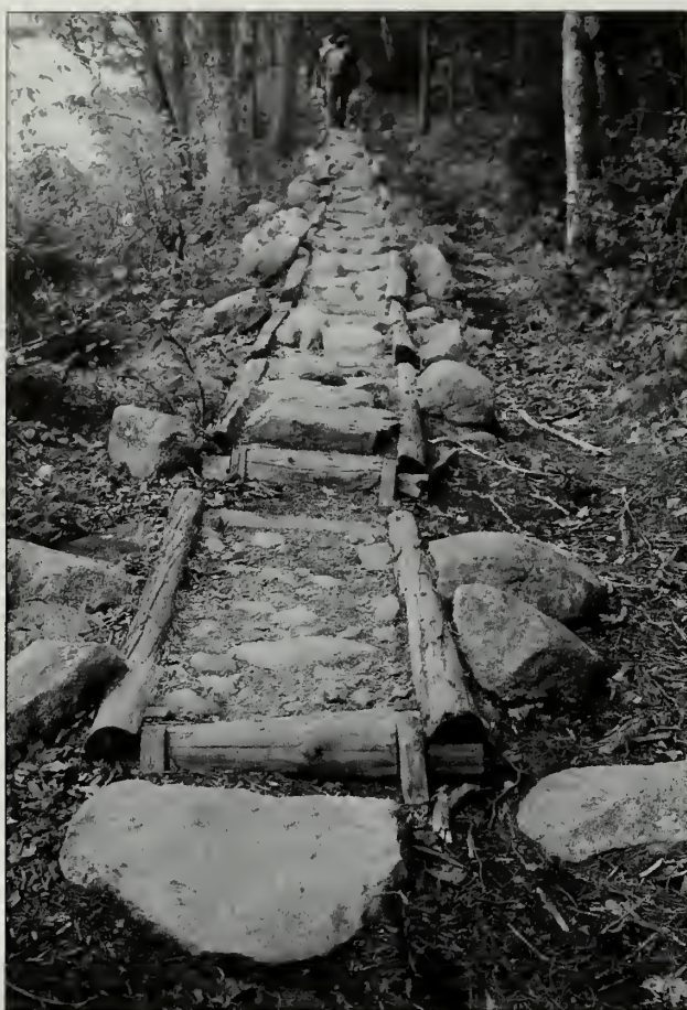
Fig. 3-15 Prior to rehabilitation, the Jordan Pond Path (#39) contained many sections of log turnpiking. Fig. 3-16 shows this same segment with the addition of new walled causeway.
