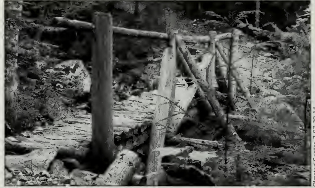
Fig. 5-37 This corduroy footbridge on the Great/Long Pond Trail (#118) was constructed in 1982, replacing an earlier CCC bridge. This new bridge is 23 feet long, 30 inches wide, and has a 3 foot railing.
