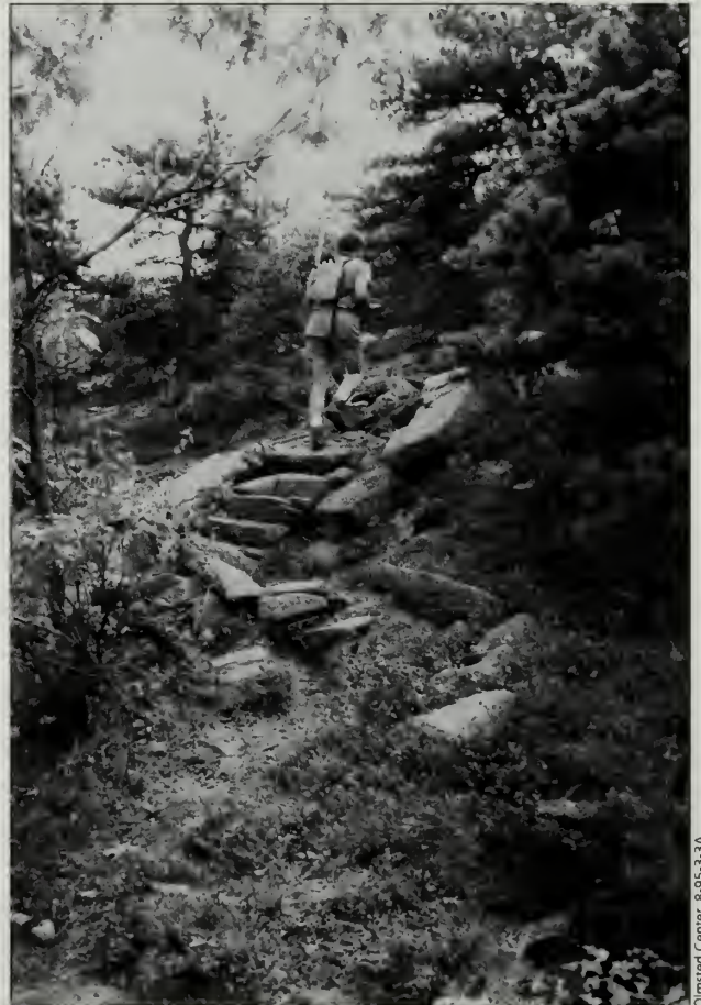
Fig. 3-50 Steps with unconstructed tread and ledge on the Upper Ladder Trail (#334).
