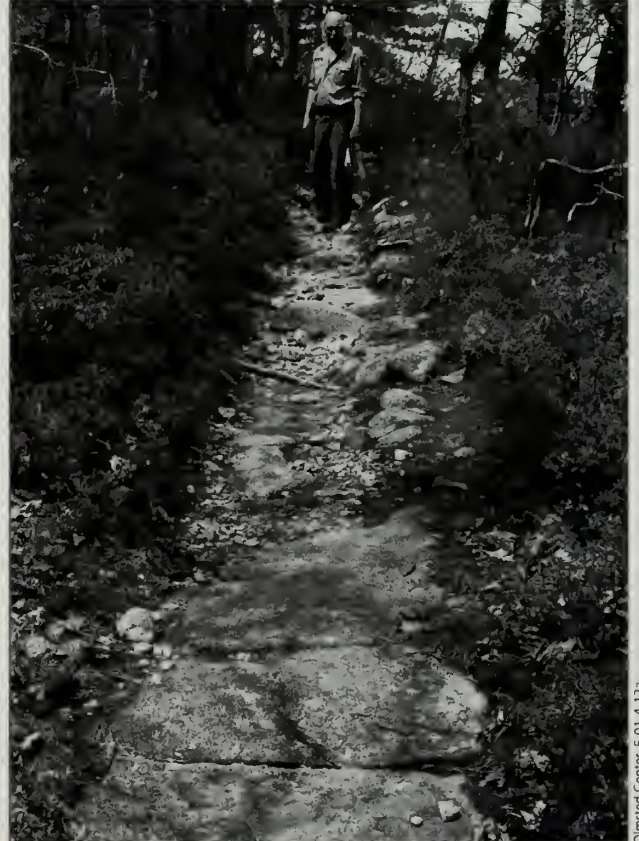
Fig. 15-8 Stone paved path with some erosion.
