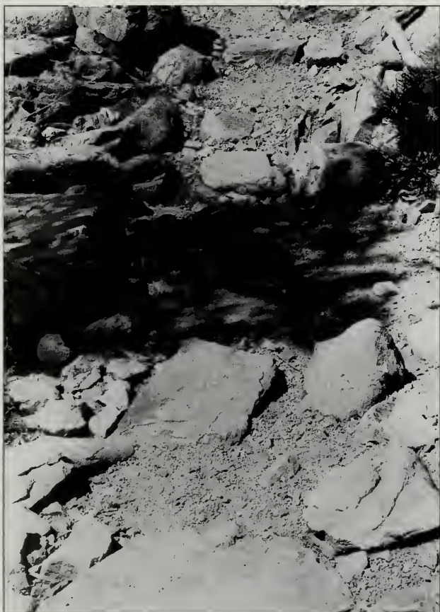
Fig. 127-14 Portion of a 50-foot section of step stones serving as stone pavement in gravel, lined with scree, constructed in 1992.
