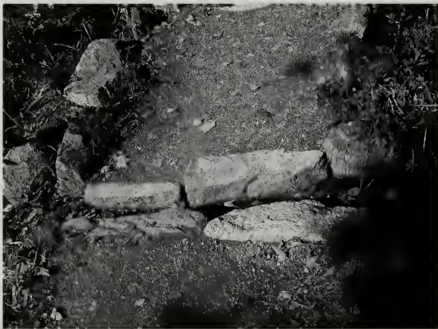
Fig. 39-27 A medium flow of water should be handled with a small open culvert. Closed culverts, although providing better visual consistency to the trail tread, would likely clog and fail regularly due to ice dams and organic debris, requiring increased maintenance.
