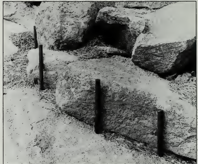
Fig. 8-14 These pins on the Beehive Path (#7) are too long and can be seen by hikers on the trail.
