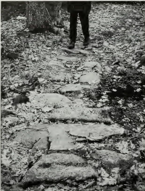
Fig. 5-54 Although these original VIS bog-style stepping stones on the Asticou Trail (#49) have settled into the ground, the irregularity of stone sizes can still be discerned.
