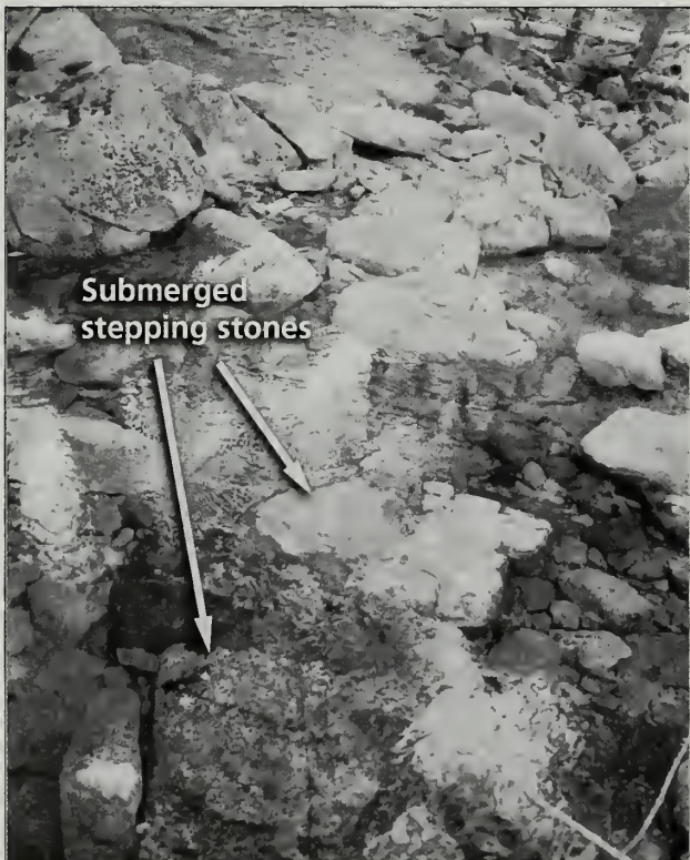
Fig. 5-65 Some of the original VIA stream-style stepping stones at this stream crossing on the Andrew Murray Young Path (#25) have sunk below the water level.
