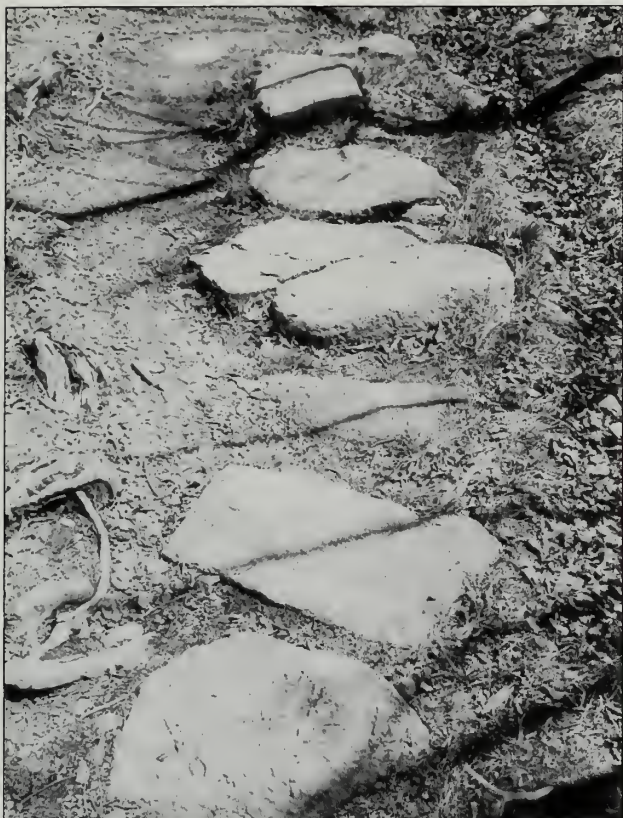
Fig. 5-56 These bog-style stepping stones on the Bowl Trail (#6) may be original VIA work.
