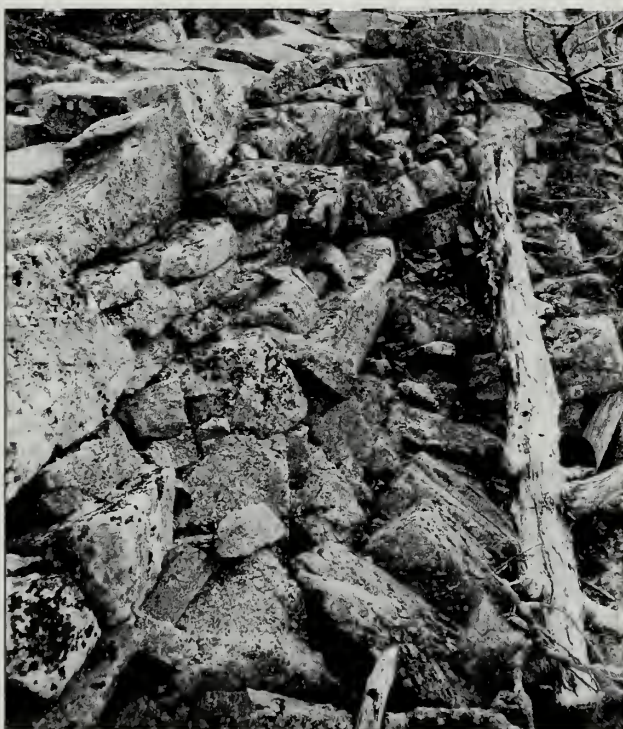
Fig. 6-32 VIA/VIS laid wall on the Beachcroft Path (#13). Stones have shifted due to "stack bonds" (unbroken, or "running joints") and areas of the wall in which three or more rocks are stacked on top of each other without overlapping the abutting stones. The weight of larger rocks on top as a coping layer is probably holding the wall together. The rough face, with some rocks jutting out, others inset, is a typical characteristic of walls on this trail as opposed to the Emery (#15) or Gurnee Path (#352) on which the walls have relatively smooth, uniform faces.
