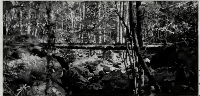
Fig. 5-27 This wooden bridge with cedar log stringers and plank decking on the Great/Long Pond Trail (#118), shown in 1968, may contain underpinnings of a CCC-era bridge.
