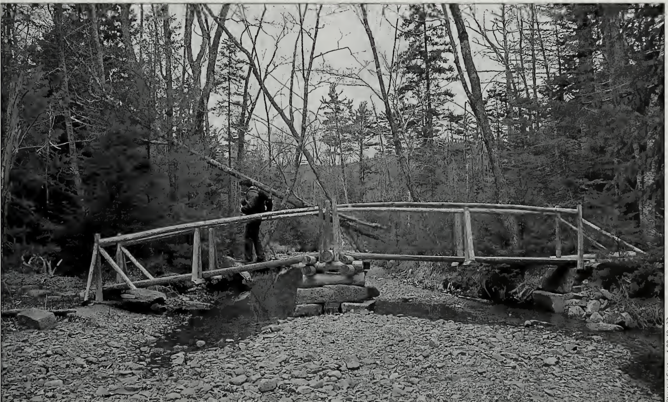
Fig. 5-62 By the 1990s, the set of VIS stepping stones shown in the previous image had been dislodged and were no longer in place. However, some of the stones were recovered from downstream and incorporated into piers and abutments for this recently built bridge. Ideally, the bridge should be removed and the stepping stones reset as they were originally.
