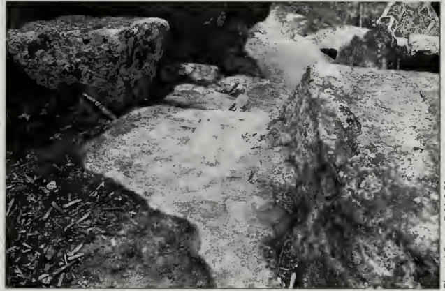
Fig. 15-20 Step cut out of ledge.
