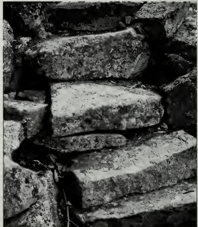
Fig. 7-27 Details of CCC steps with shims on the Perpendicular Trail (#119).
