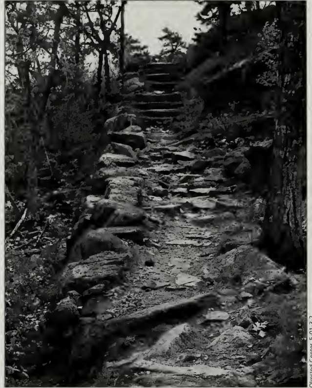
Fig. 15-6 The same view in 2001 as Fig. 5-1 in the 1920s, but with gravel surface washed away.
