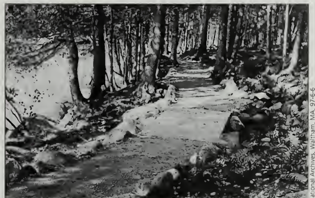
Fig. 5-51 Small CCC corduroy bridge on the Great/Long Pond Trail (#118) in 1935. The delicate style, similar to earlier VIA/VIS work, complements the gravel tread and coping stones.
