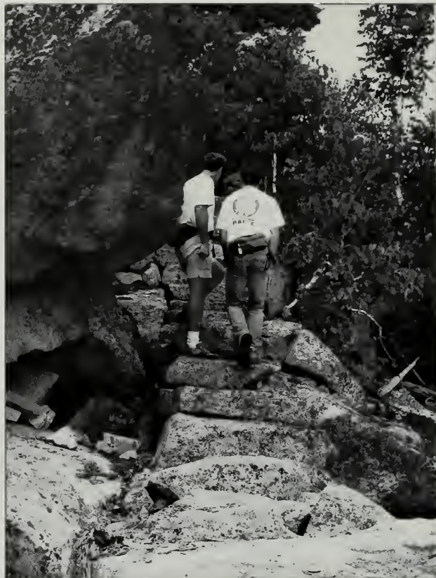
Fig. 349-15 Path passing beside jutting boulder, raised with retaining wall and blocking.
