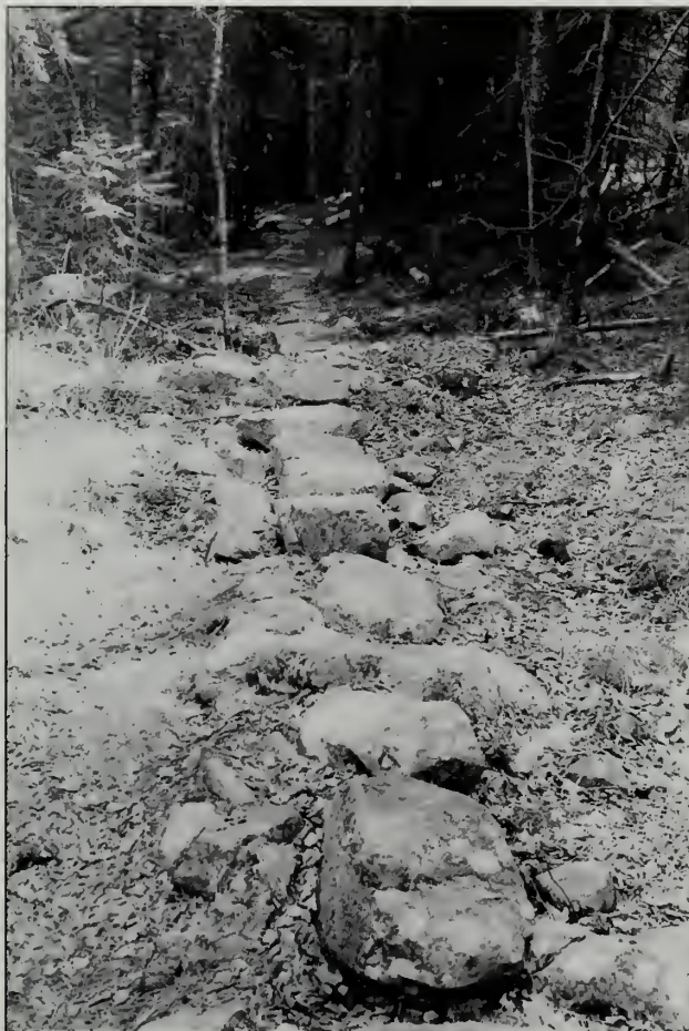
Fig. 5-53 It is unknown whether these stepping stones on the Eagle Lake Trail (#42) are original VIA/VIS work, but they reflect the style of VIA/VIS stepping stones used in boggy areas.
