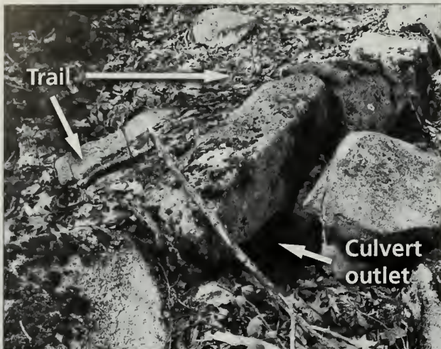
Fig. 349-12 Graveled-over culvert located 60 feet from the trail beginning.
