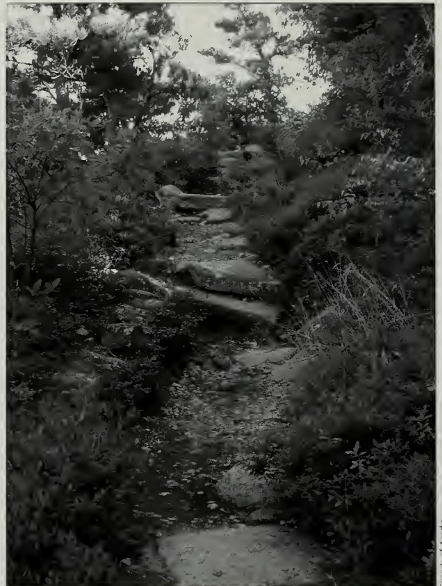
Fig. 15-13 Eroded section with collapsed steps that need to be rebuilt.
