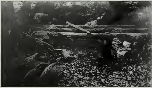
Fig. 5-29 A 1930s view of construction of a CCC corduroy bridge shows the installation of the stone abutments and three log stringers.
