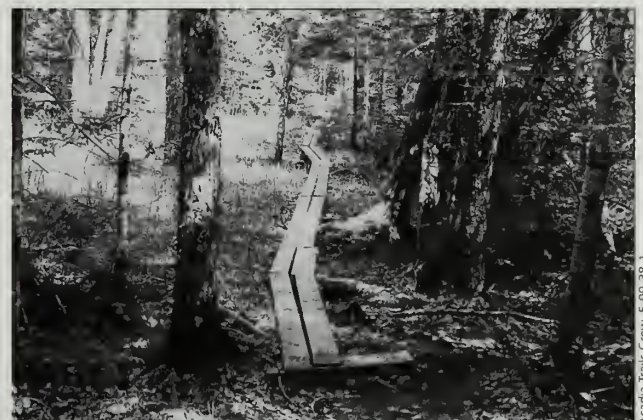
Fig. 5-4 This 1990s plank bogwalk (possibly 2-by-6-inch lumber) on private land on the Jordan Stream Path (#65) may be Seal Harbor VIS construction.
