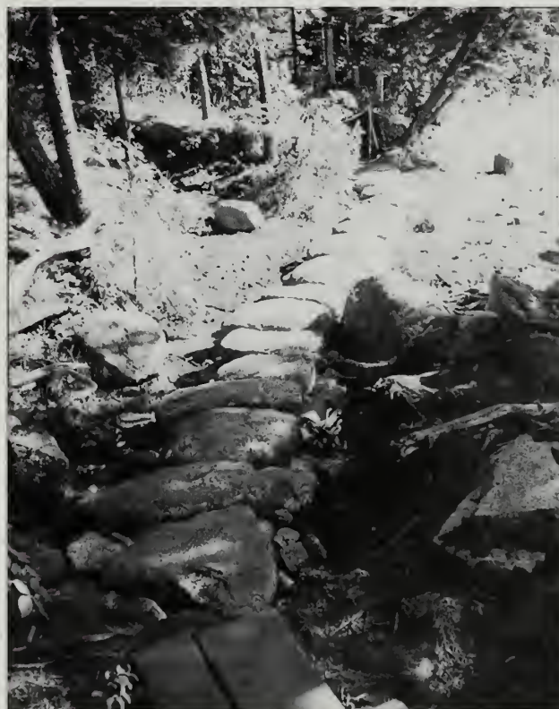
Fig. 5-70 Replacement bog-style stepping stones installed by NPS in 2002. Note the even curve, level, flat tops, and crushed rock.
