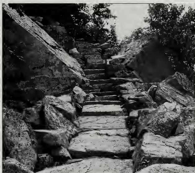
Fig. 7-17 A narrow stone staircase between sections of stone pavement on the Beachcroft Path (#13).
