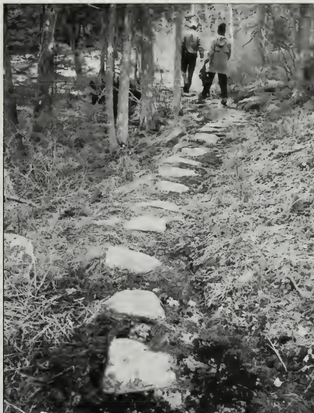
Fig. 5-57 These bog-style stepping stones on the Canon Brook Trail (#19) are in the VIA/VIS style, but it is not known if these are original trail features.
