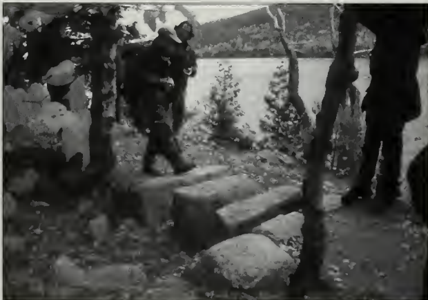
Fig. 39-28 This step stone culvert was installed on a newly rehabilitated section of trail to handle a heavy water flow.
