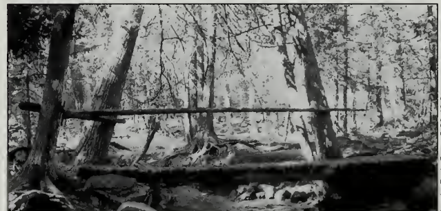
Fig. 5-28 This corduroy bridge on the Lower Hadlock Trail (#502) has a single wooden railing nailed to adjacent trees. It was constructed in the 1990s by the Northeast Harbor VIS.
