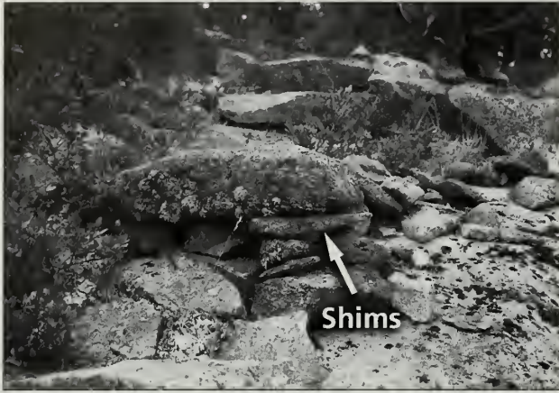
Fig. 7-5 These steps on the Upper Ladder Trail (#334) contain exposed shims. Their use may have contributed to the deterioration of these Bates-style steps since shims are generally not locked in place and are often dislodged.
