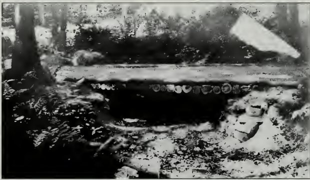
Fig. 5-30 The completed corduroy bridge with log curbs and gravel over the decking photographed in the 1930s. Its smaller scale is typical of CCC work on the west side of the island.
