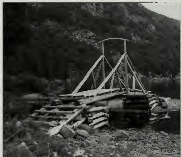
Fig. 39-9 This wooden bridge was constructed in 1983 and reinstalled on wooden crib piers in 1987.
