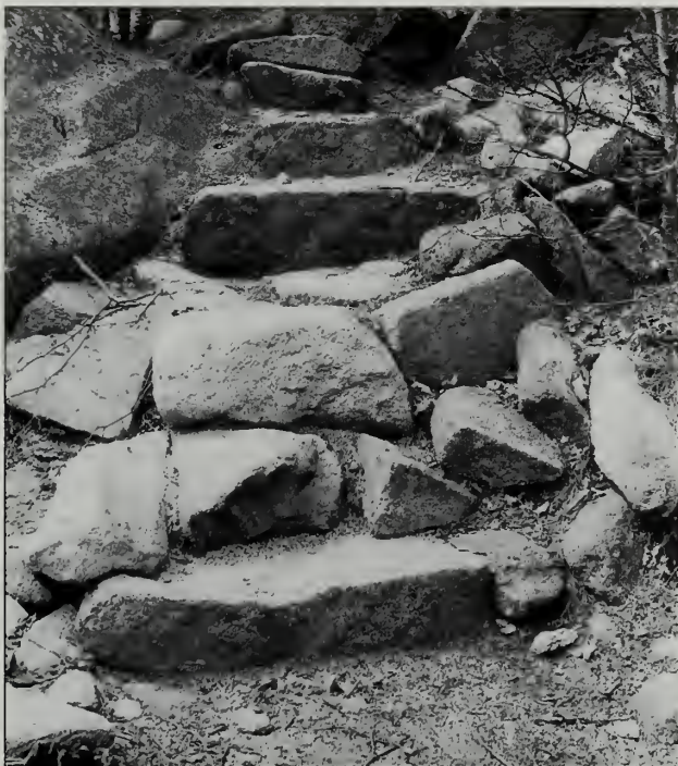
Fig. 7-21 A partially reconstructed stone staircase on the Beehive Trail (#7). The rehab is misfitting, as the odd-shaped stones of random sizes on the lower part of the staircase do not resemble the historic, evenly laid rectangular stones on the upper part of the staircase.
