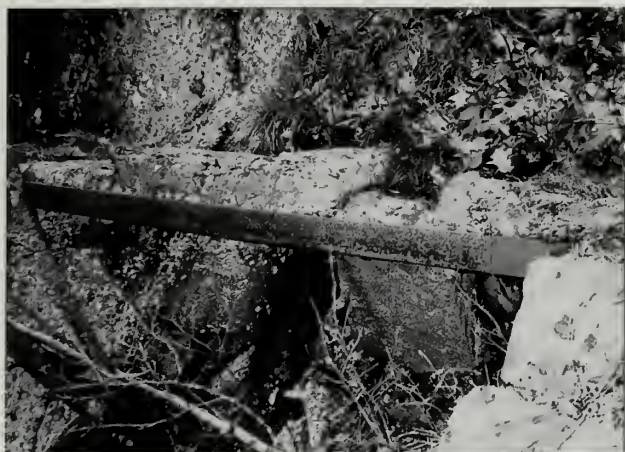
Fig. 8-16 Side view of iron bridge surfaced with flat stones on the Cliff Path (#347).
