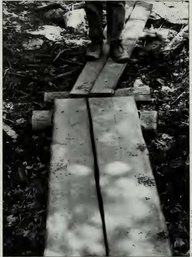
Fig. 39-29 Bogwalk should be uniform in length and width. For example, this bogwalk on the western side of Jordan Pond is not of uniform width at the joint, making it more difficult for hikers to walk along safely.
