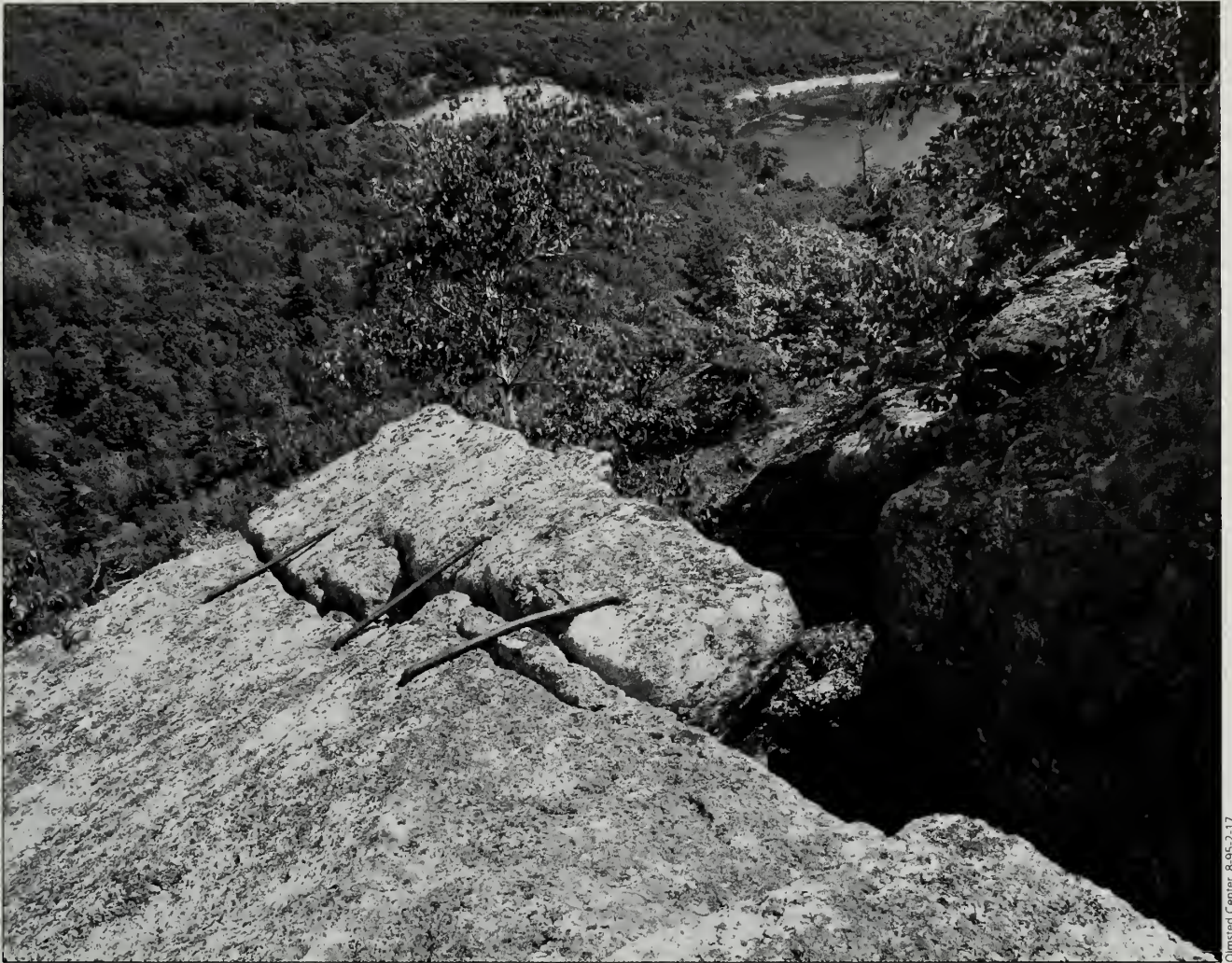
Fig. 8-1 Iron pins hold an overhanging boulder at Sieur de Monts Crag on the Emery Path (#15).
