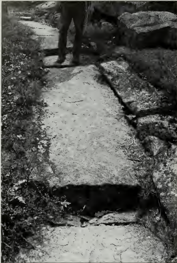
Fig. 15-9 Stone paved trail with capstone culvert in good condition.
