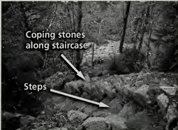
Fig. 6-19 The CCC regularly used coping stones along stairways on the Perpendicular Trail (#119). They serve several purposes, including adding structural stability to the staircase and providing a definitive boundary for the trail edges.
