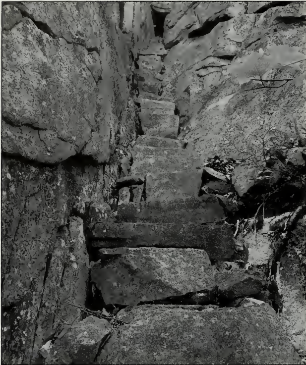
Fig. 7-23 Brunnow-style stone steps on the Champlain East Face Trail (#12).
