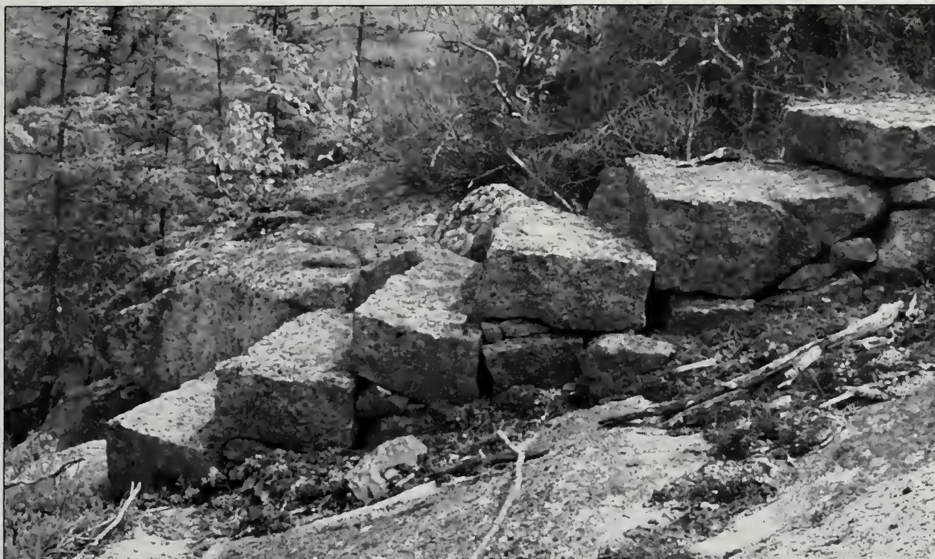
Fig. 7-14 Dorr-style stone staircase on ledge rock on the upper section of the Homans Path (#349).
