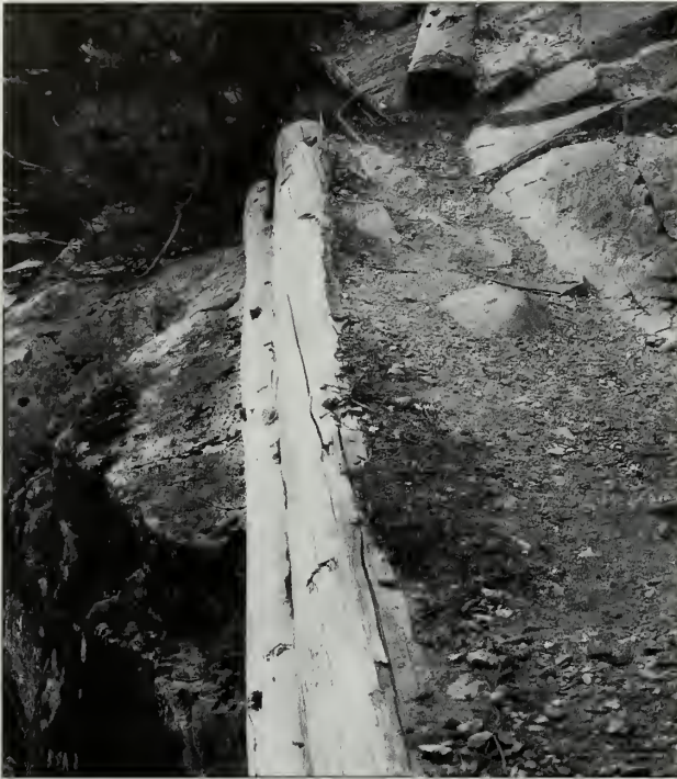
Fig. 6-40 Log features, like this log retaining wall on the Long/ Great Pond Trail (#118), have been introduced as a quick and cheap alternative to stone retaining walls, although they are not historically appropriate for the system.
