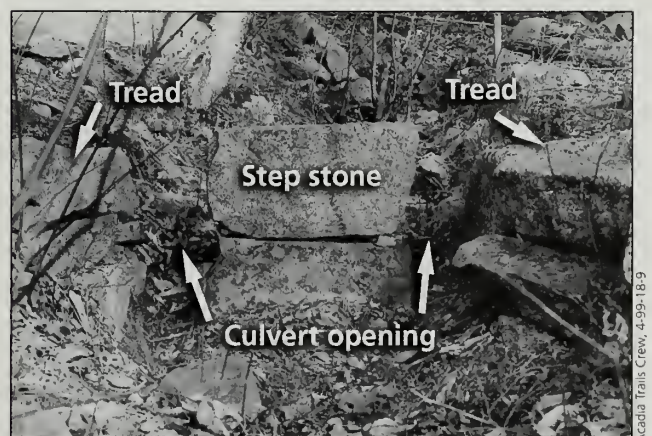
Fig. 4-6 A stepstone culvert on the Kane Path (#17).
