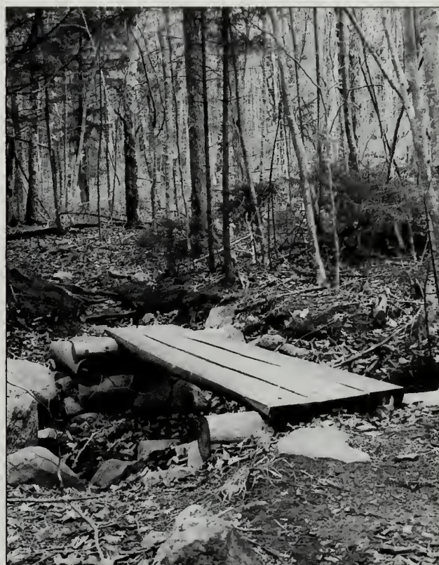
Fig. 5-9 A bogwalk bridge on the Jordan Pond Carry Path (#38).
