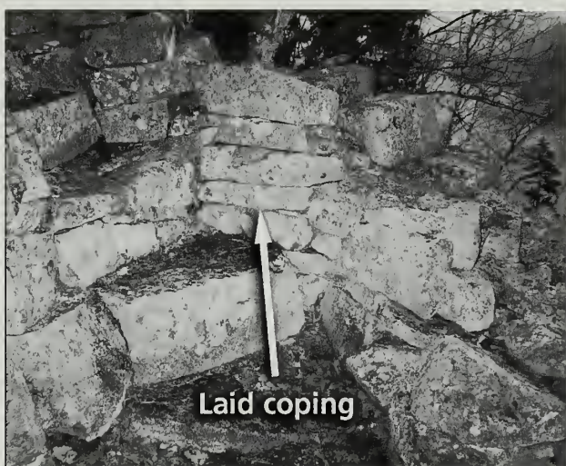
Fig. 6-12 Laid coping wall on the Perpendicular Trail (#119).
