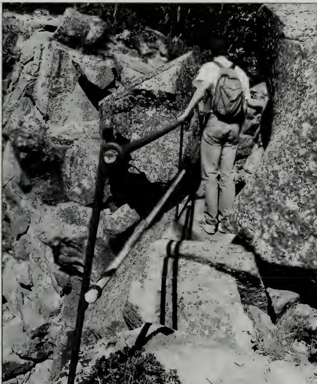
Fig. 8-4 Railing supported on stanchions on the Orange and Black Path (#348).
