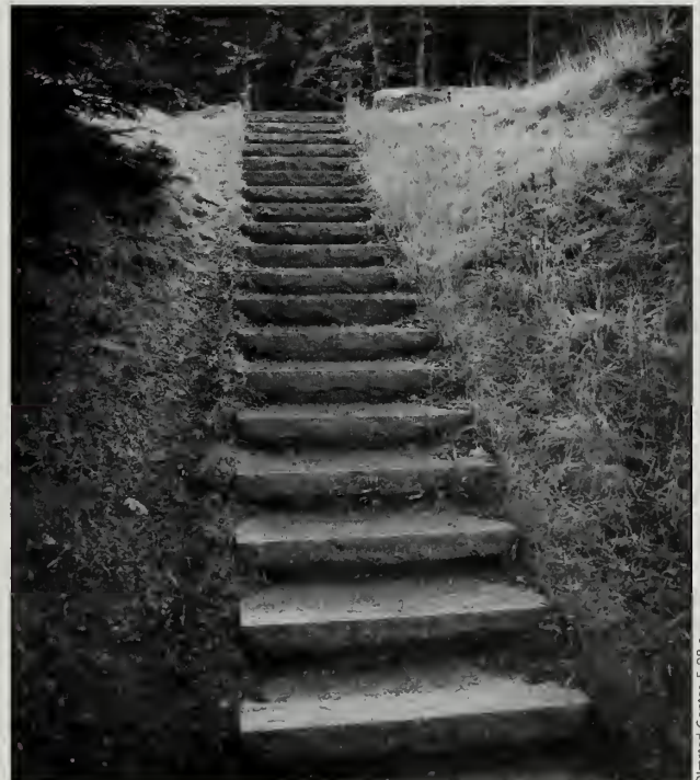
Fig. 7-41 These stairs from the Park Loop Road to Western Point, south of Blackwoods Campground, are too uniform and are out of place in the Acadia trail system.
