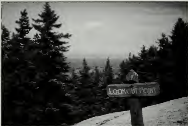
Fig. 9-31 A 1958 photo of a 1930s CCC trail sign at Lookout Point on the Mansell Mountain Trail (#115). The sign is nailed to a notched post that was stained brown and cut with a conical top. The sign had tapered ends and was also stained brown with chiseled letters painted yellow.
