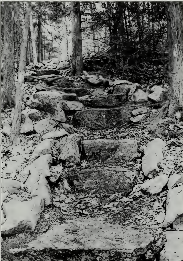
Fig. 7-25 These CCC steps on the Acadia Mountain Trail (#101) contain consistent sizes of stones. The AMC scree installed later along the trail edges has altered the historic character.
