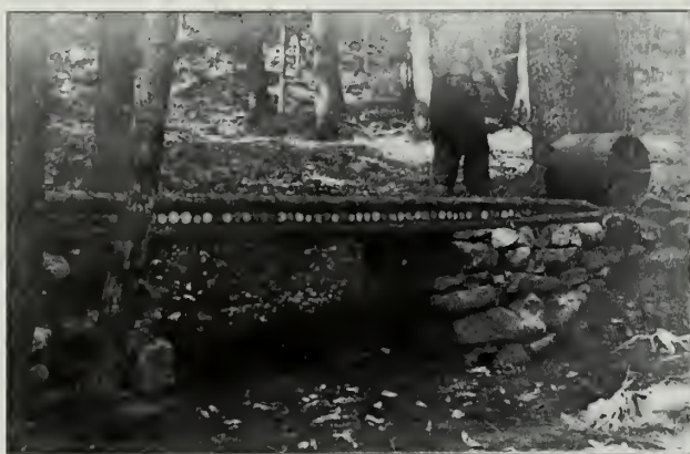
Fig. 5-47 A CCC worker rolls gravel tread on a corduroy bridge on the Stratheden Path (#24) in the 1930s. Notice the stone abutments, corduroy decking, and curbrails, common features on many of the gravel surfaced bridges.
