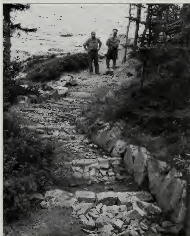
Fig. 6-6 Checks, wall, and rubble infill in place.
