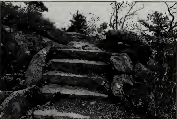
Fig. 15-18 Stone steps with coping stones and retaining wall behind.
