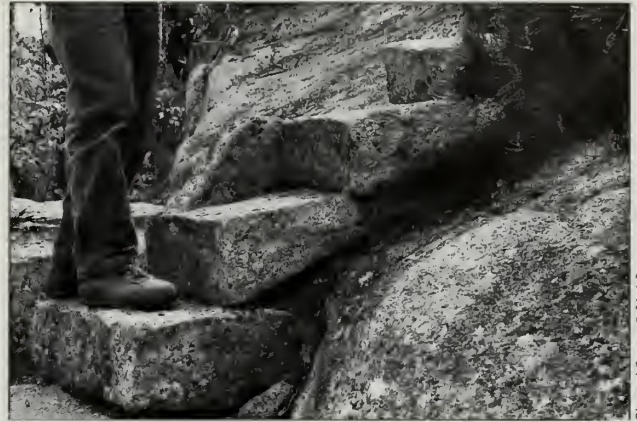
Fig. 15-19 Slab-laid steps.
