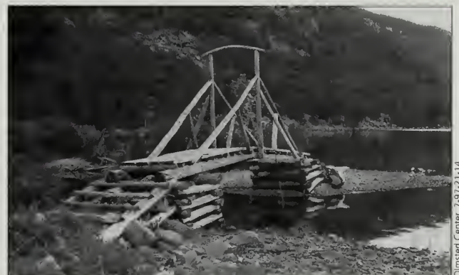
Fig. 5-46 This wooden bridge was constructed in 1983 by NPS crews on the Jordan Pond Loop Trail (#39) at the north end of the pond.
