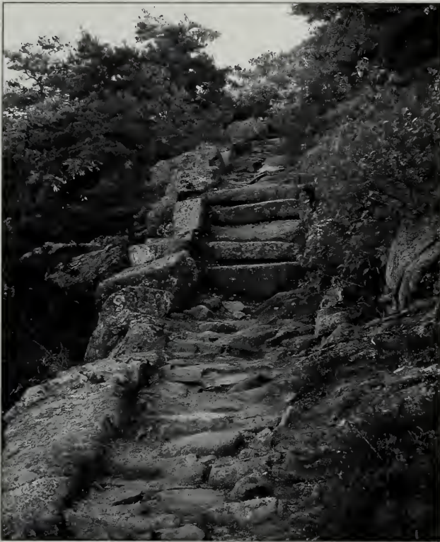
Fig. 15-17 Stone steps with coping, some steps and coping stones have slipped.
