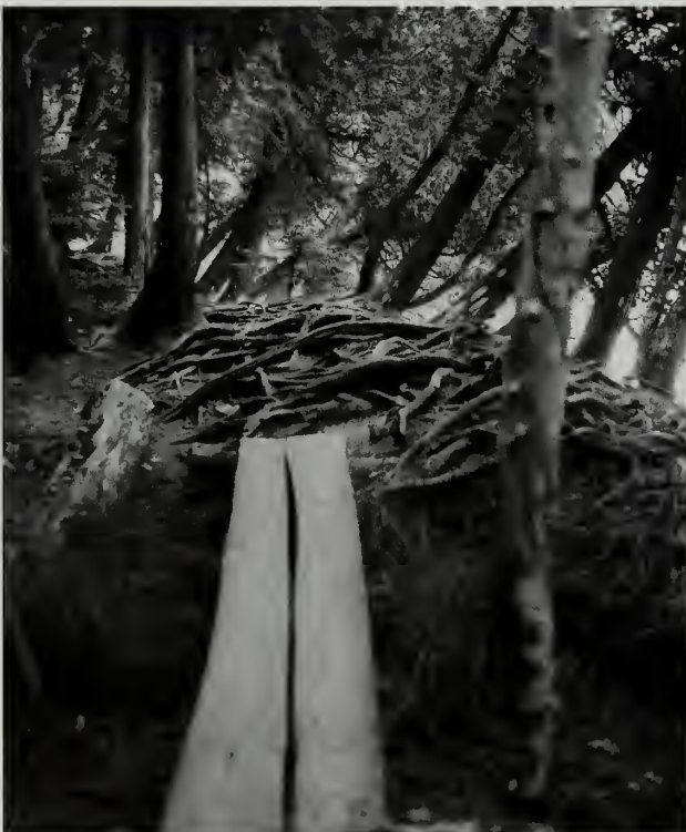
Fig. 5-6 Bogwalks are an effective, easily constructed way to provide stable tread over wet or exposed root areas such as on the west side of the Jordan Pond Loop Trail (#39).
