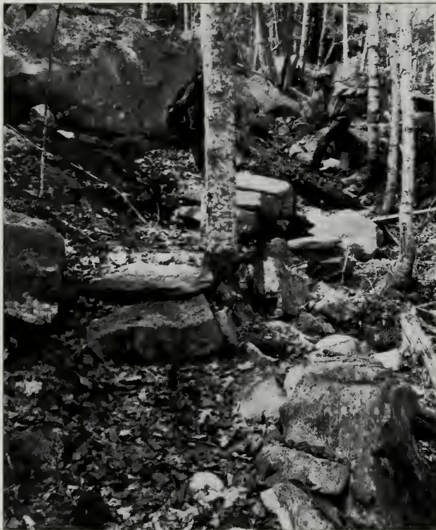
Fig. 349-7 Approximately 230 feet from entrance, a 24-foot section of collapsed tread and uprooted trees shows the abandoned condition of some trail segments.
