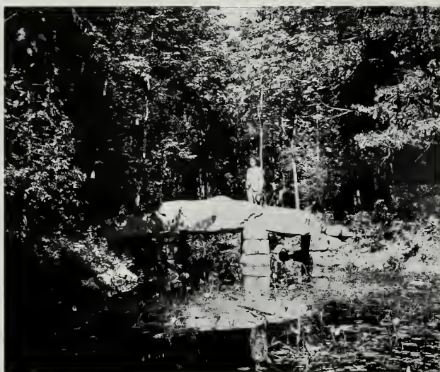
Fig. 5-48 The Kane & Bridgham Memorial Bridge was constructed between 1926 and 1929 at the outlet of Lakewood in Bar Harbor. Designed by noted landscape architect and summer resident Beatrix Farrand, the bridge consisted of large stone slabs set on stone piers. Photograph circa 1932.
