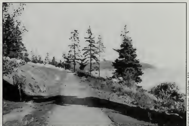
Fig. 3-23 CCC-constructed causeway on the Ocean Path (#3), shown in the 1930s.
