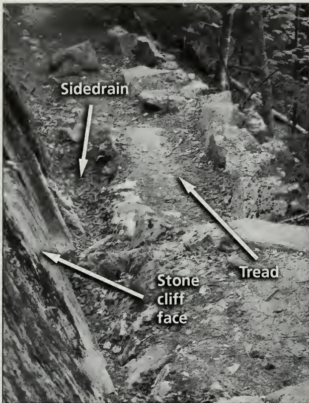
Fig. 4-32 A walled side drain along a stone cliff face on the Perpendicular Trail (#119).
