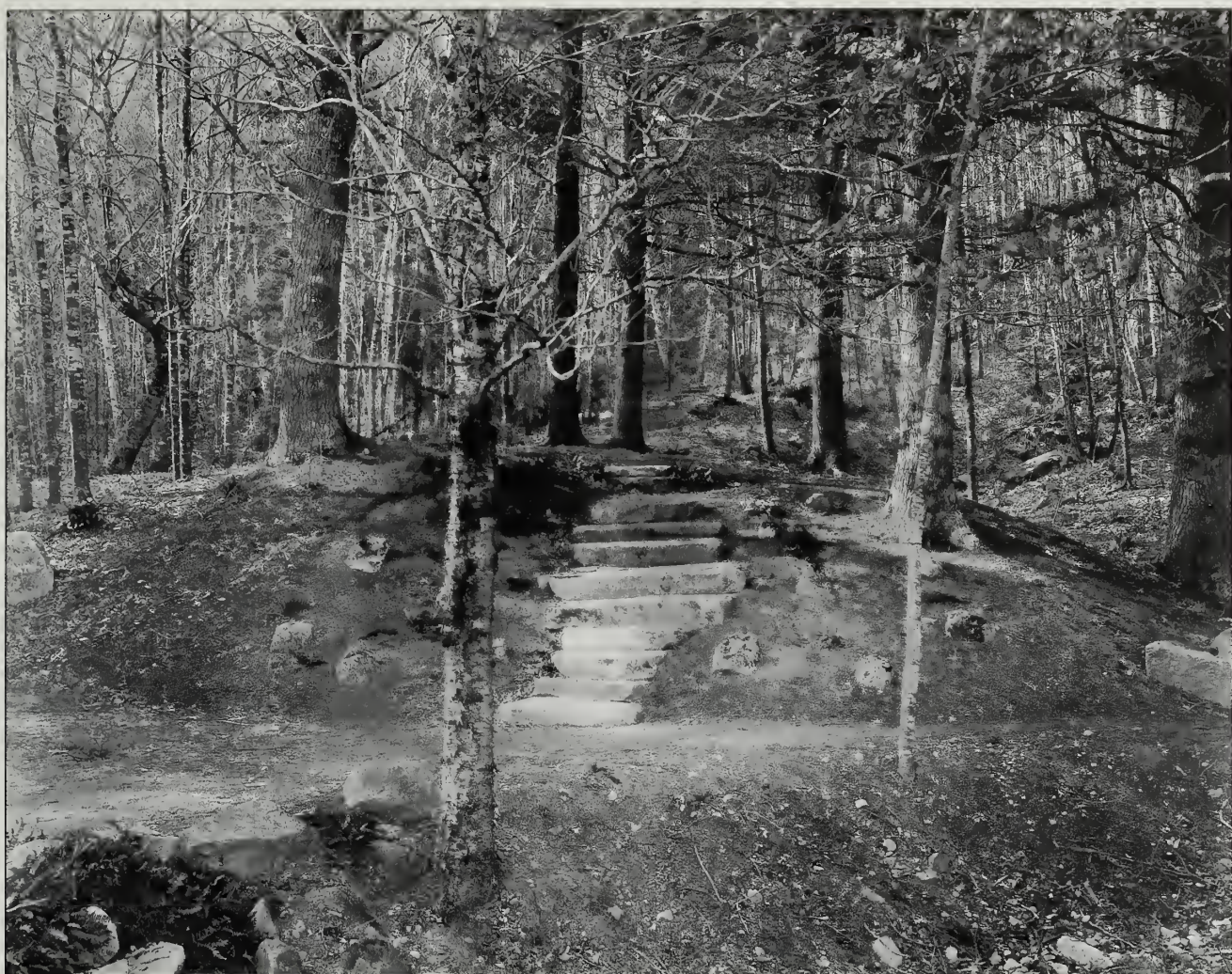
Fig. 7-1 This staircase at the trailhead of Kurt Diederich's Climb (#16), circa 1916, is one example of the highly crafted stone step work that exists on Acadia's trails.
