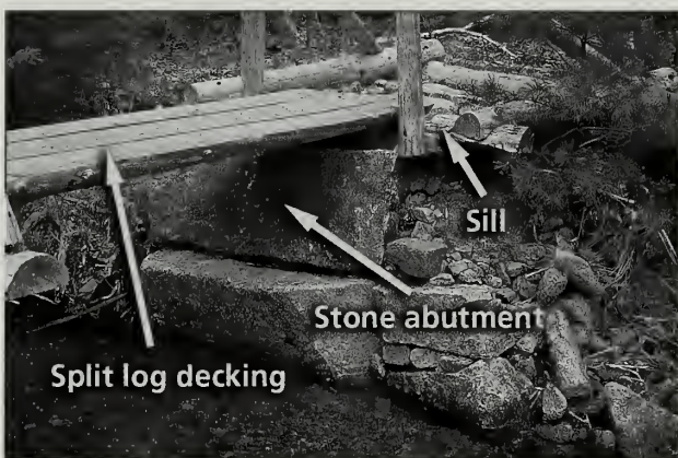
Fig. 5-17 Plank bridge over Harbor Brook on the Asticou Trail (#49).
