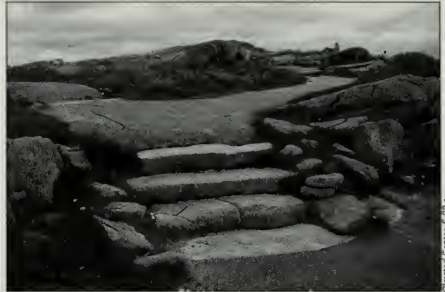
Fig. 7-24 Stone steps and asphalt pavement on the Cadillac Summit Loop Trail (#33).
