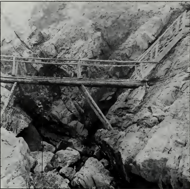
Fig. 5-23 A bridge of cut boards and rough-hewn logs, shown in 1908, along the rocks near Seal Harbor built by the Seal Harbor VIS, circa 1908.
