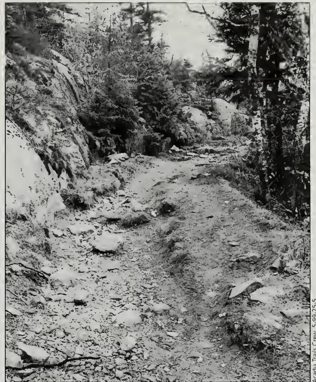
Fig. 6-3 This section of the Beech Mountain Loop Trail (#113) is a perfect candidate for the use of checks to reverse ongoing erosion and tread loss.
