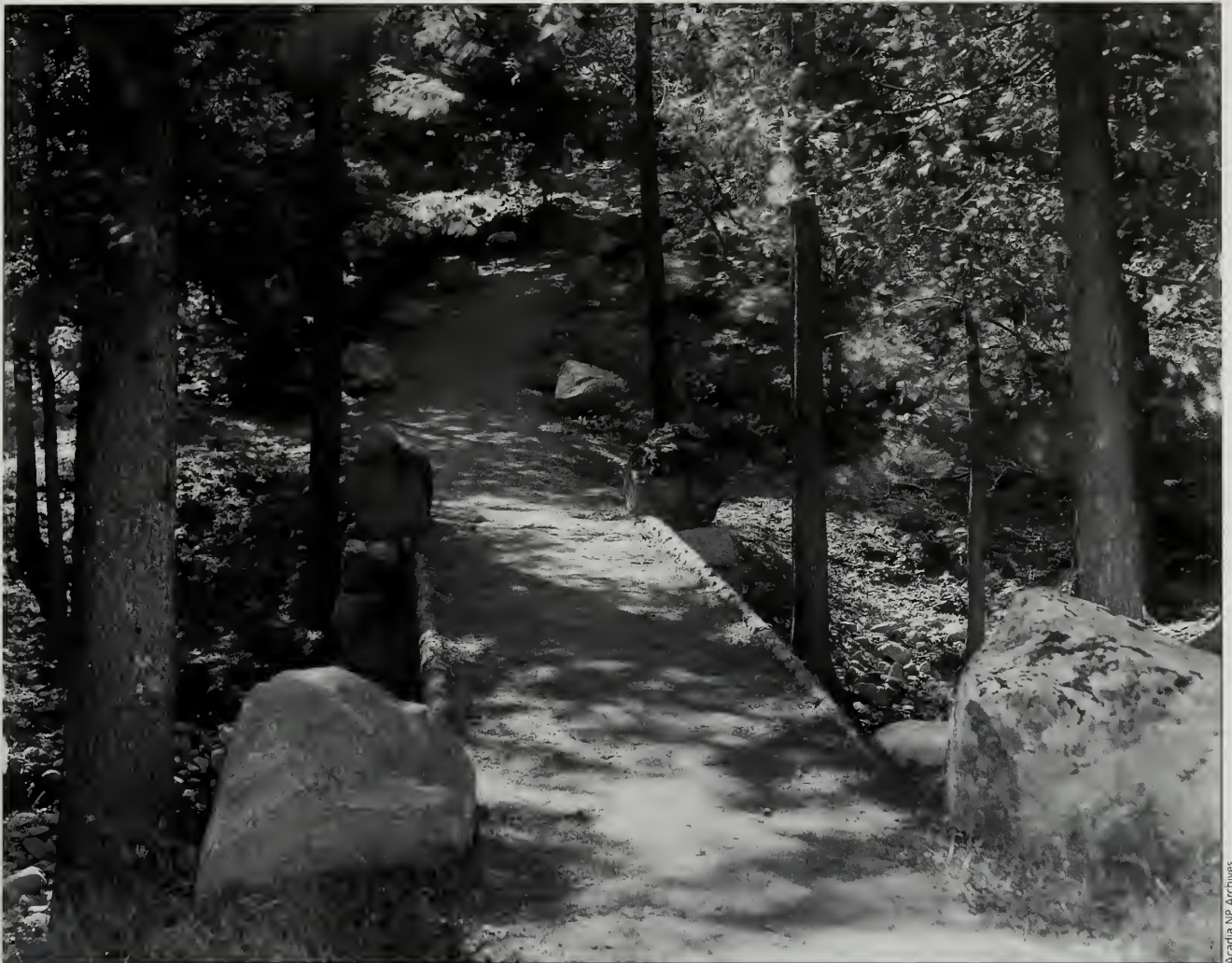
Fig. 5-1 The Bar Harbor VIA constructed many small gravel-surfaced bridges as stream crossings in the Sieur de Monts area like this one across Kebo Brook on the Stratheden Path (#24), circa 1916.
