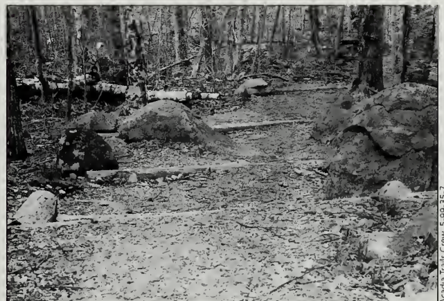
Fig. 4-40 A series of log water bars on the Jordan Pond Carry Spur (#40).
