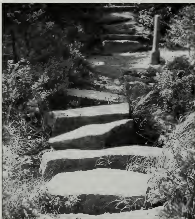
Fig. 5-60 A contemporary view of the Tarn stepping stones, looking west toward trailhead of Kurt Diederich's Climb (#16).
