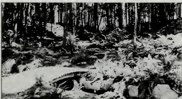
Fig. 5-40 This historic image shows an arched CCC corduroy bridge near the Cold Brook Fish Hatchery on the Great/Long Pond Trail (#118) soon after construction in 1935.
