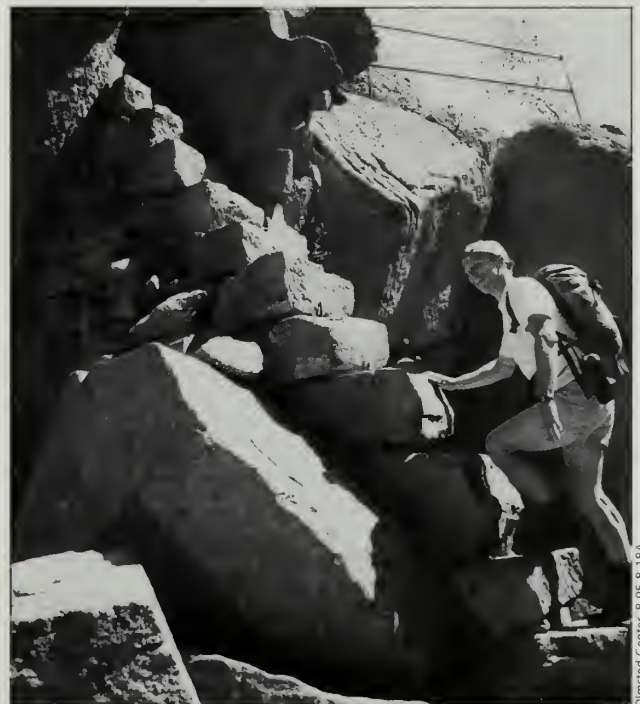
Fig. 7-22 Brunnow’s “Hanging Steps” on the Orange and Black Path (#348). Steps are pinned in the front and middle. Note the exposed retaining wall under the upper steps.
