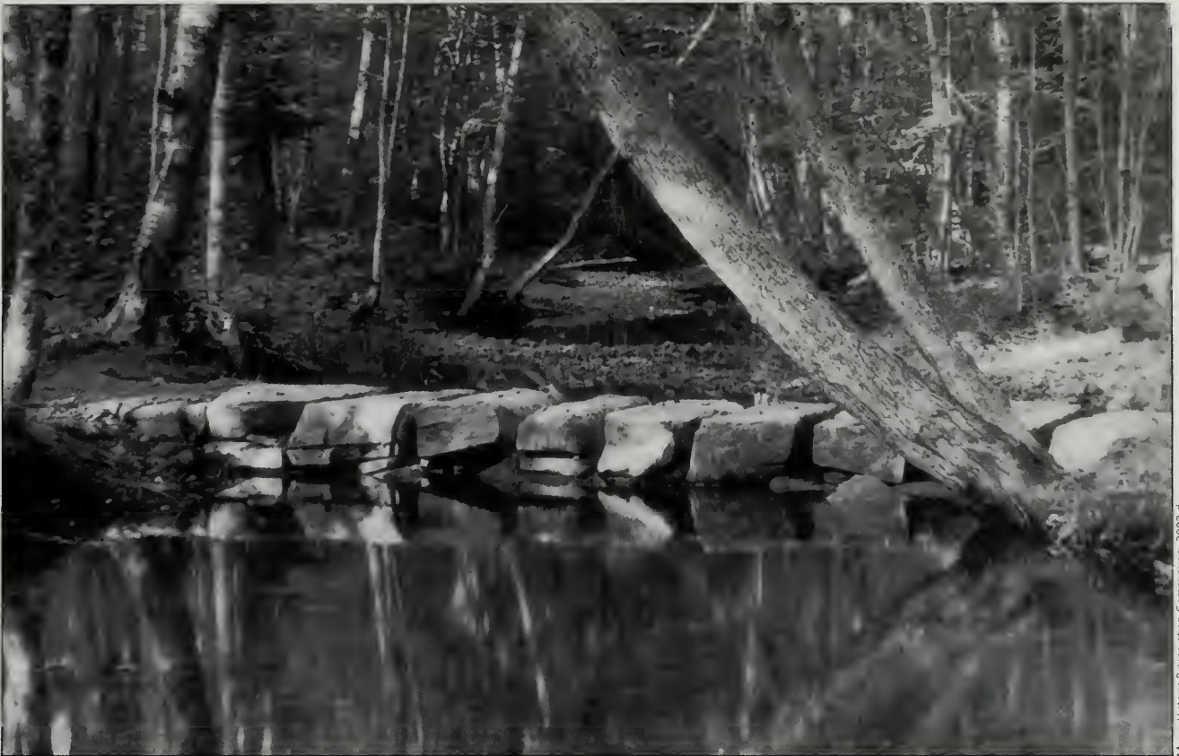
Fig. 5-61 This circa 1920 postcard view shows original stream-style stepping stones on the Asticou Trail (#49) crossing Harbor Brook. These stones probably date to the trail's improvements by the Northeast Harbor VIS and Seal Harbor VIS in the early 1900s.
