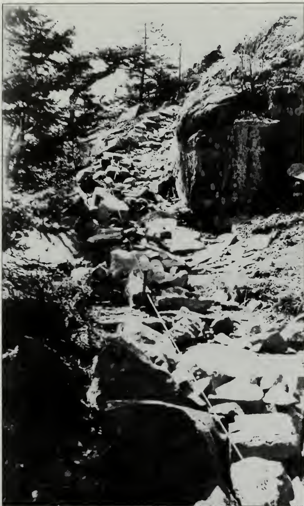
Fig. 1-13 The CCC used string to lay out the route and finished grade of their new trails, as shown at the construction of the Ocean Path (#3) at Otter Cliffs.
