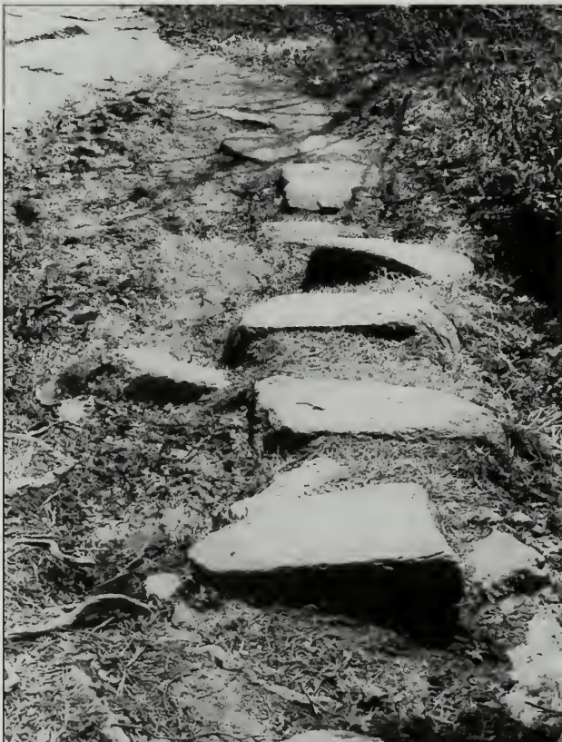
Fig. 5-55 These VIA bog-style stepping stones are located on the Gorham Mountain Trail (#4).
