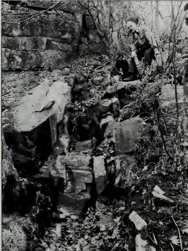
Fig. 48-8 Ascending ledges below shoulder of Sargent Mountain. Section in poor condition needs steps and checks.
