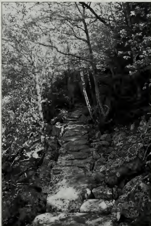
Fig. 3-39 This talus pavement on a section of Kurt Diederich's Climb (#16) is one of the fine examples of VIA/VIS stone pavement in the trail system.
