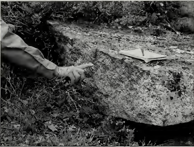
Fig. 349-19 Hand showing drill marks on a nearby ledge where steps were quarried.
