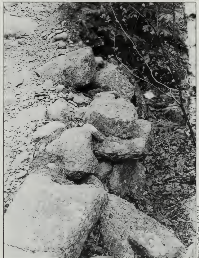
Fig. 6-38 Original Mission 66 rubble retaining wall on the Beech Mountain Loop Trail (#113).
