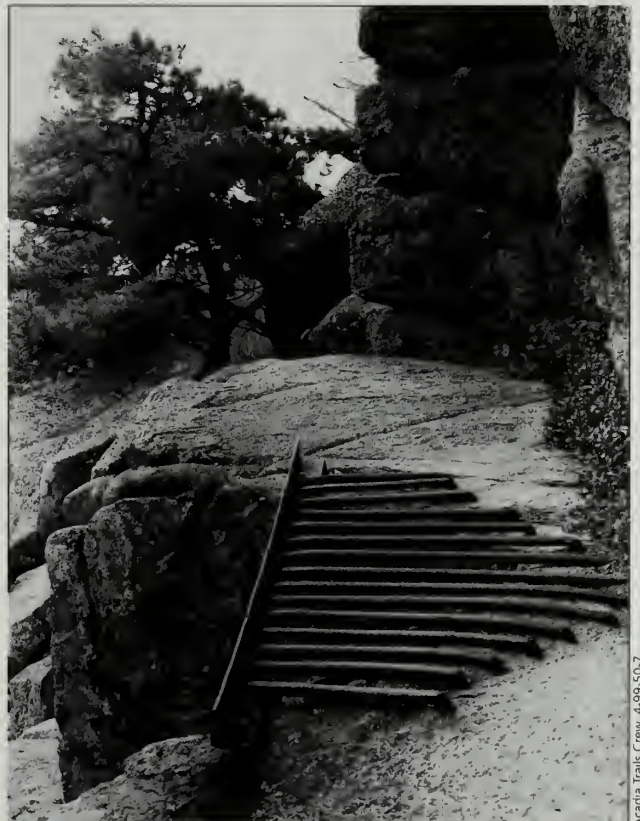
Fig. 8-6 An iron bridge on the Beehive Trail (#7).
