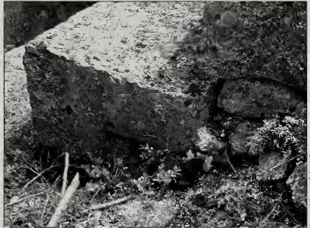
Fig. 349-22 Detail of a pinned step on the Homans Path.
