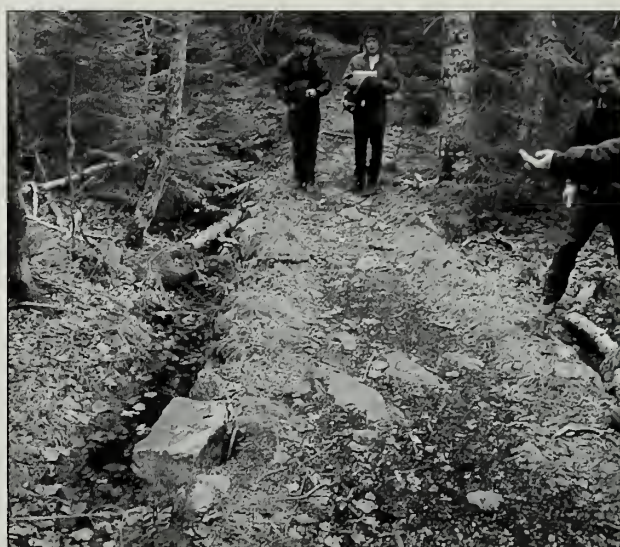
Fig. 3-17 This walled causeway on the Asticou Trail (#49) is still extant and in relatively good condition over one hundred years later.
