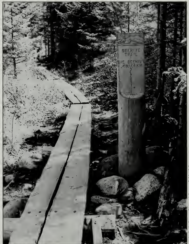
Fig. 5-7 Bogwalks are often installed to protect fragile vegetation, like this section surrounding The Bowl on the Beehive Trail, West (#8).
