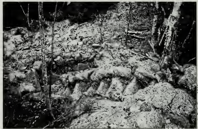
Fig. 7-26 Highly engineered CCC switchbacks of uniform steps cutting through a talus slope on the Perpendicular Trail (#119).
