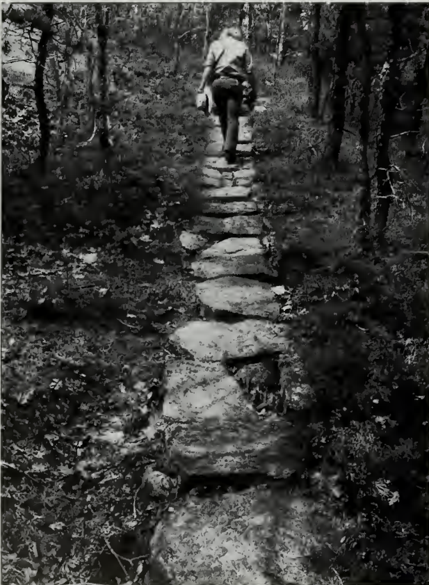
Fig. 15-7 Stone paved trail in good condition.
