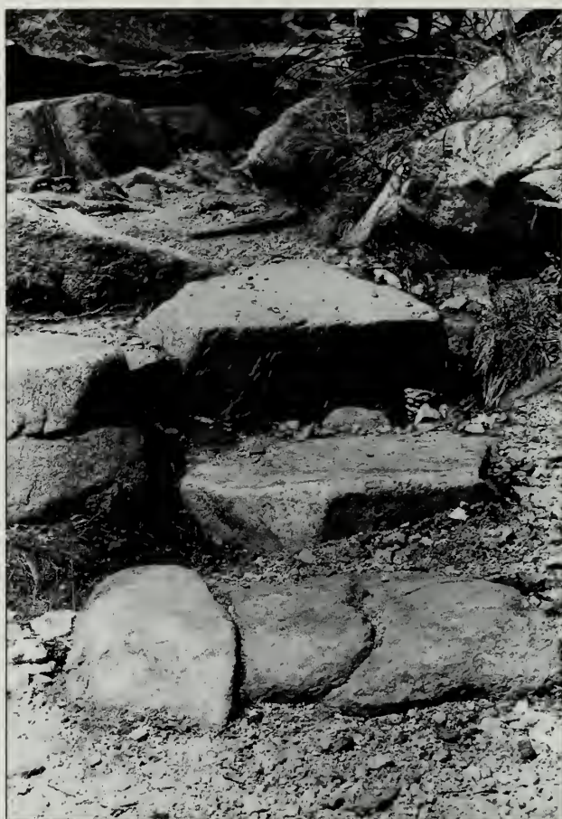
Fig. 127-13 Slab laid steps built in 1991 of local basalt.
