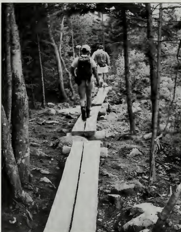
Fig. 1-17 Reroute of flooded segment of the Bowl Trail (#6) shown in Fig. 1-16 located farther away from the edge of the pond. Bogwalk was installed to traverse wet, muddy areas. However, this feature is not in keeping with the historic stepping stones that are present on other sections of this trail.
