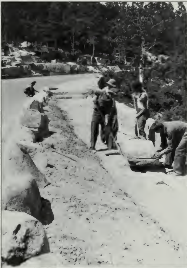
Fig. 6-22 Coping stones newly installed by the CCC and Rockefeller's road crew between Ocean Drive and the Ocean Path (#3), circa 1934.
