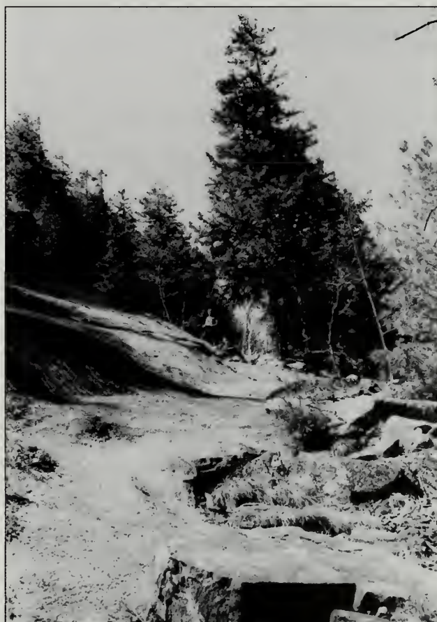
Fig. 3-52 Unconstructed tread on the Norumbega Mountain Trail (#60) has continued to erode from increased use, leaving the trail corridor more than 10 feet wide in some places.
