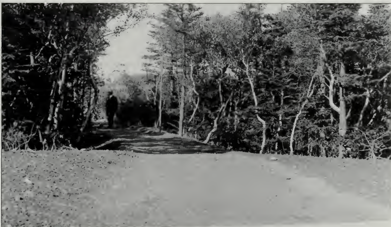
Fig. 3-30 Newly installed CCC gravel, photograph showing completed work in the 1930s.
