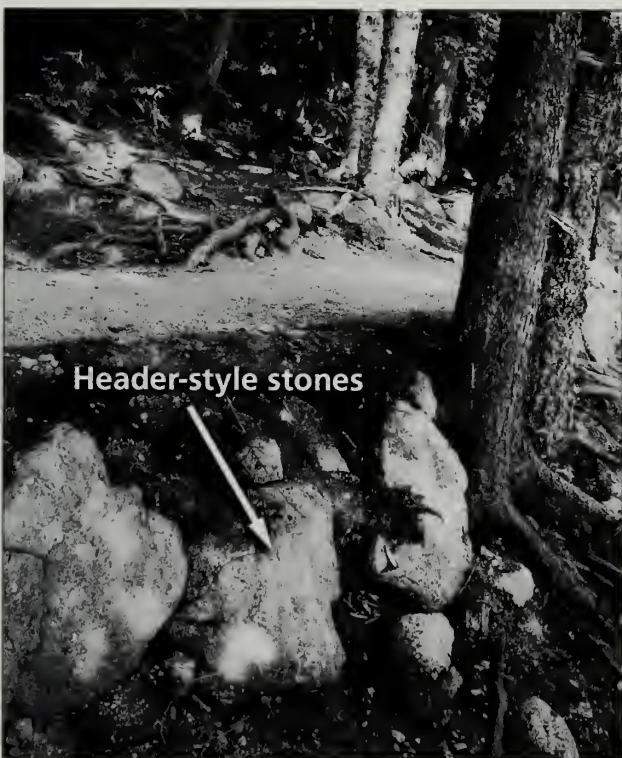
Fig. 6-30 New crush wall constructed by NPS in 2002 through heavily rooted area on the west side of the Jordan Pond Path (#39).
