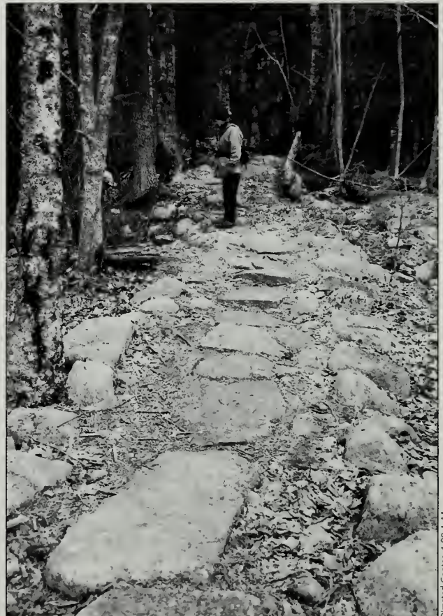
Fig. 6-18 Coping stones are used sparingly on the Andrew Murray Young Path (#25). Here they are used in conjunction with stone pavement.
