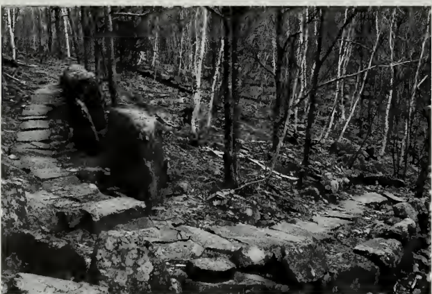
Fig. 3-38 Tread pavement through a wooded section of the Beachcroft Path (#13).
