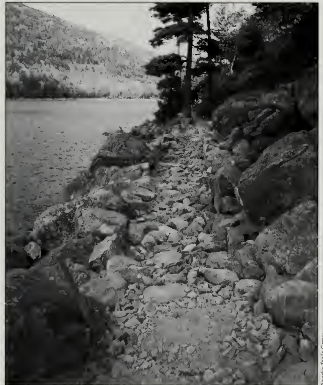
Fig. 39-16 The same view as Fig. 39-5 taken in 2001 showing NPS rehabilitation in progress. The base is in place, but the final application of gravel tread has not been completed.
