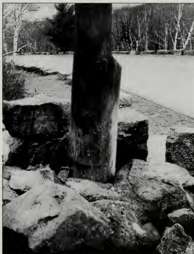
Fig. 8-37 Pinning technique used to deter sign vandalism on signpost at the Bear Brook Trail trailhead (#10).
