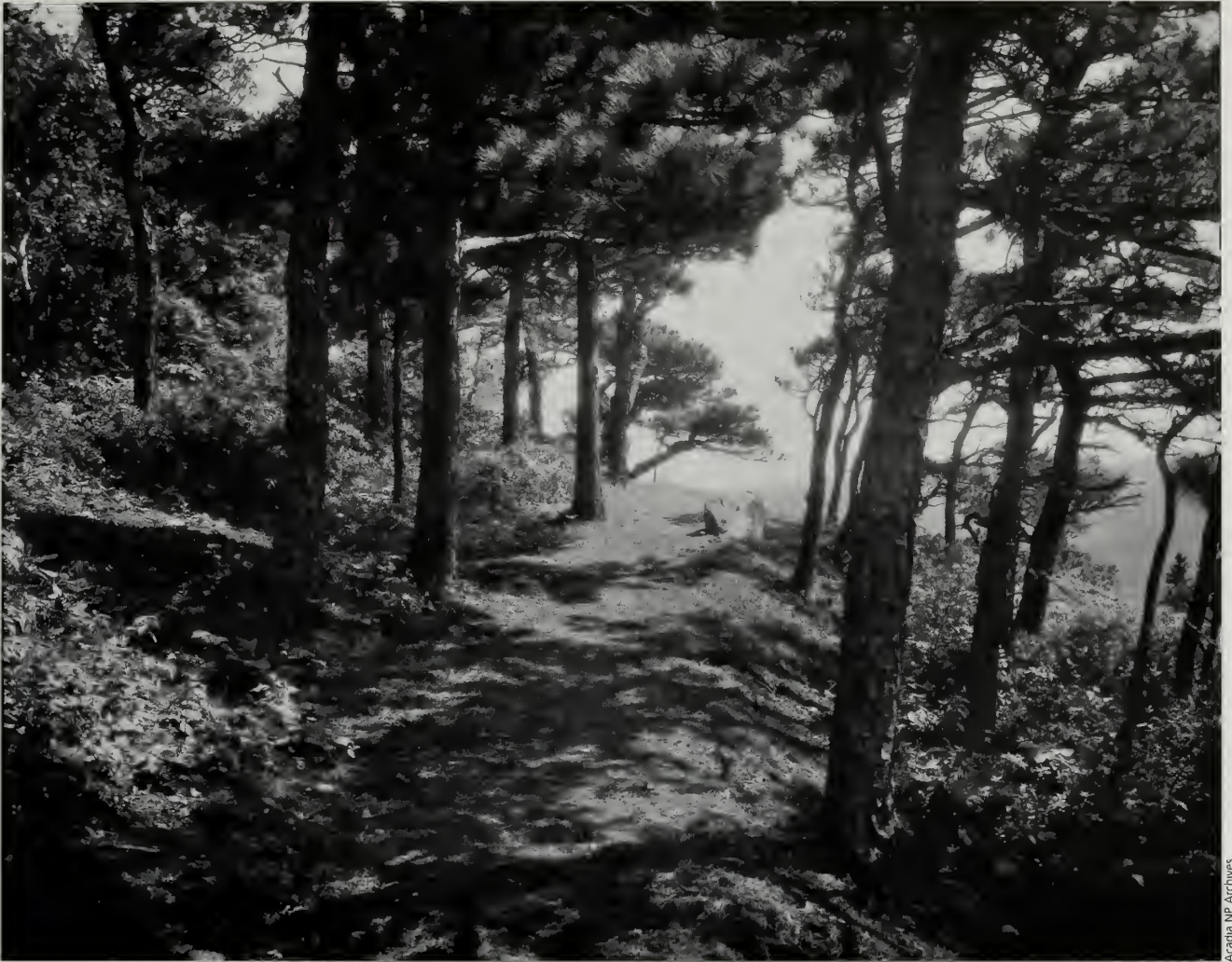
Fig. 3-1 This circa-1916 photograph of a bench cut on the Beachcroft Path (#13) illustrates how the treadway enhances the overall trail character. Near the trailhead, the trail is highly crafted with almost continuous stone pavement along its sidehill route. As it approaches Huguenot Head and winds through a grove of trees, the character changes to a woodland walk, emphasized by a treadway surfaced with pine needles and other organic material.
