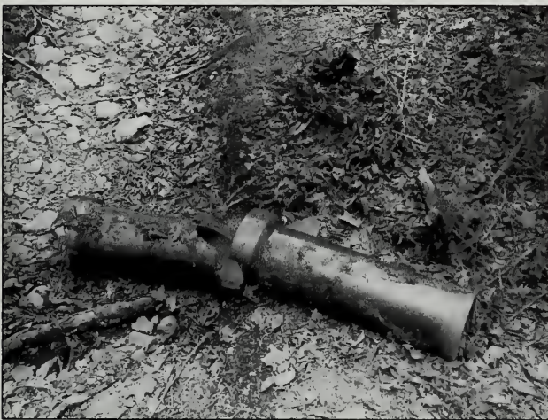
Fig. 4-8 A defunct VIA/VIS vitrified clay pipe culvert on the Seaside Path (#401), south of the Stanley Brook Bridge.
