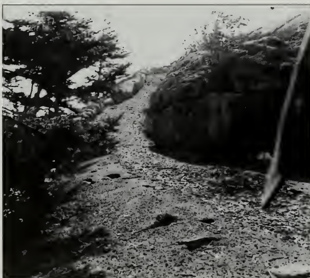
Fig. 1-14 Completed section of path shown in Fig. 1-13. The CCC emphasis on maintaining an even grade is evident in this newly completed section of the Ocean Path (#3) at Otter Cliffs.
