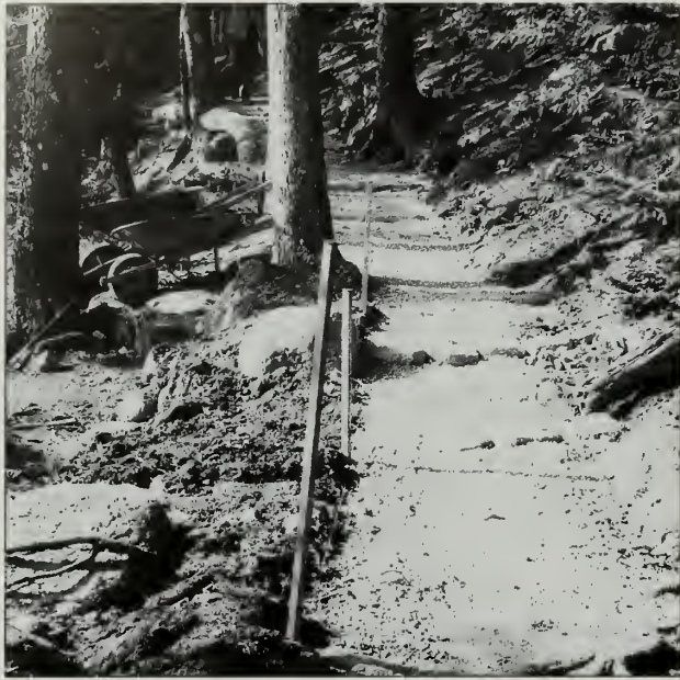
Fig. 39-26 Wall crib and checks installed by NPS in 2002 in same section shown in Fig. 39-25.
