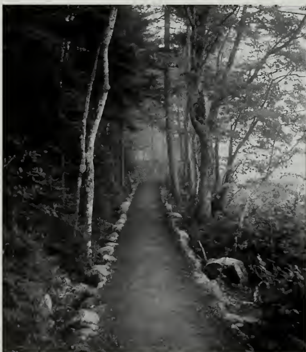
Fig. 3-16 Recently rehabilitated walled causeway on the Jordan Pond Path (#39) in section formerly treated with log turnpiking.
