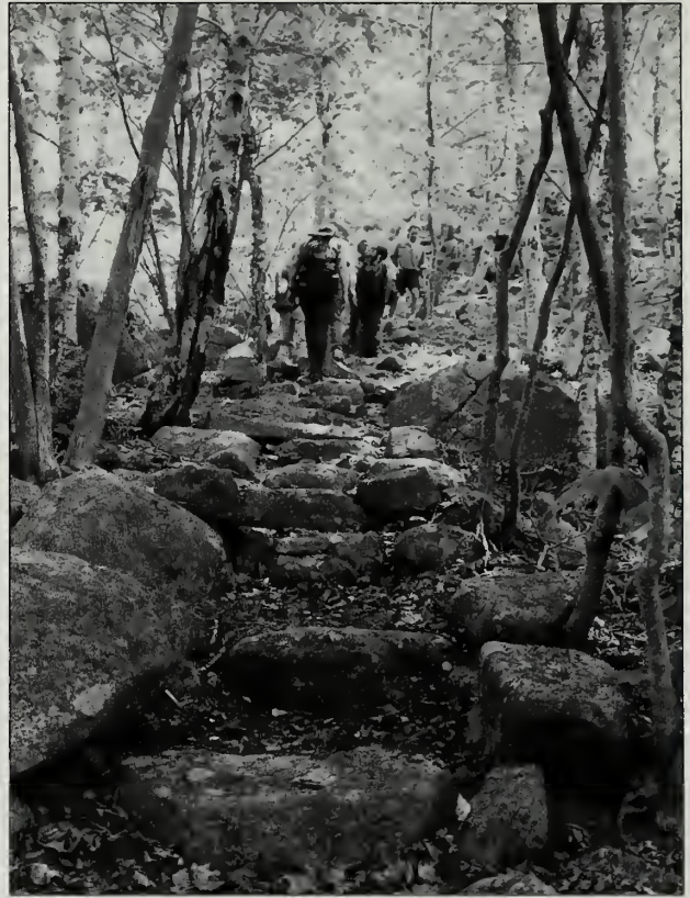
Fig. 7-8 Bates-style steps on the Goat Trail (#444).
