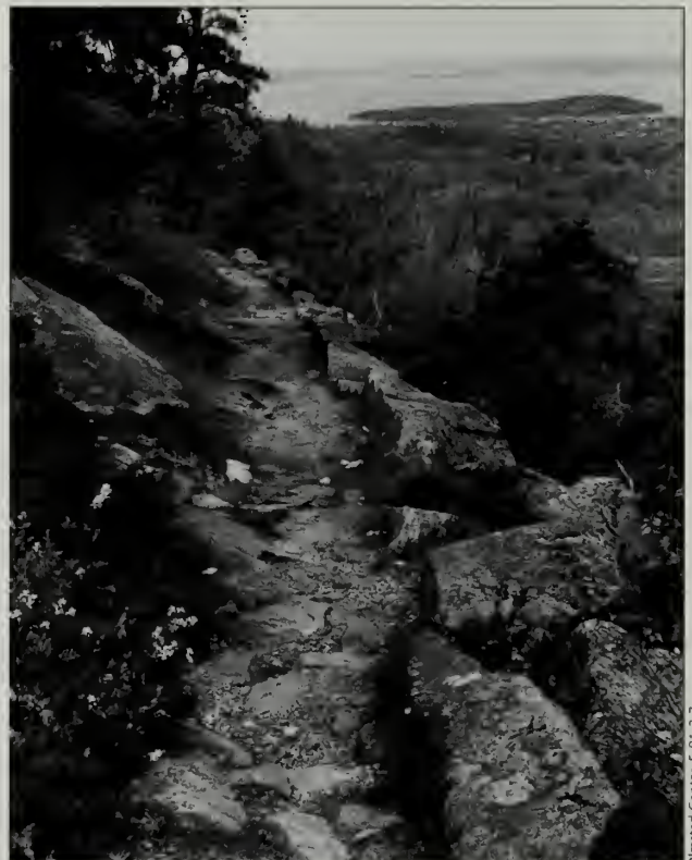
Fig. 15-15 Very large coping stones are used along this area of exposed ledge rock to retain the tread. Some of the stones have slipped.
