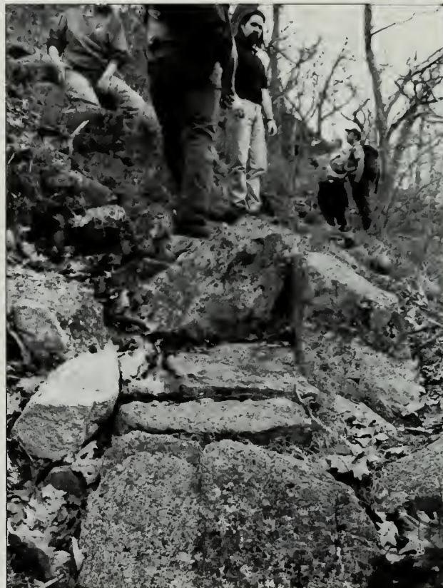
Fig. 48-15 A short run of coping stones, steps, and stone pavement on ledges in poor condition.
