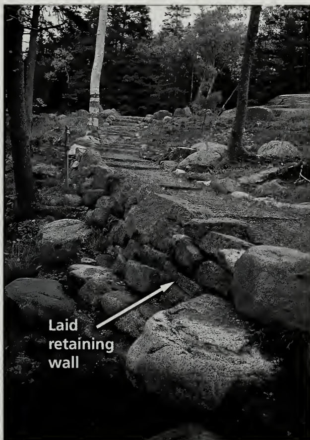
Fig. 6-24 A recently constructed laid retaining wall on the Ocean Path (#3) at Otter Point.
