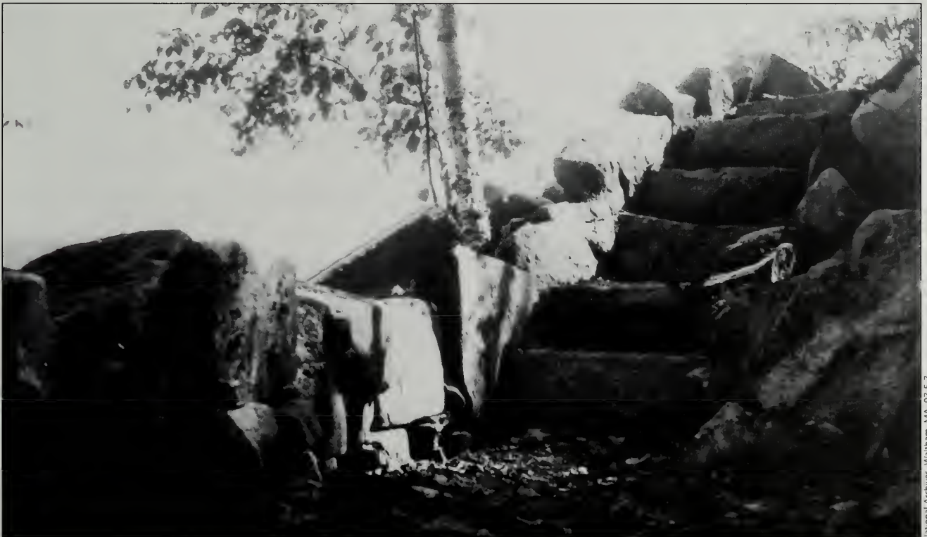
Fig. 6-20 Coping stones define the edge of this small CCC staircase on the Perpendicular Trail (#119), circa 1934.
