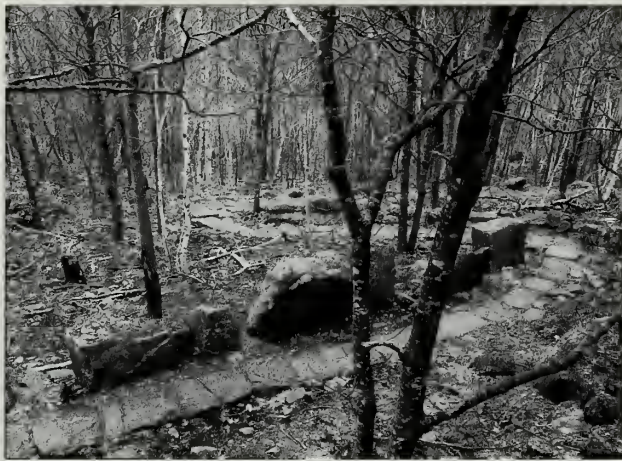
Fig. 6-16 Large coping stones are used along the lower section of the Beachcroft Path (#13) to help define the trail sides.
