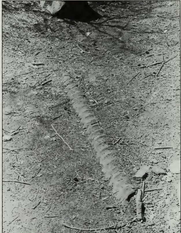
Fig. 127-10 This original pipe culvert is in poor condition. It is exposed and clogged with no side ditches available for outlets.
