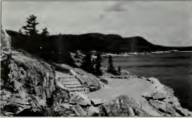
Fig. 1-23 The CCC used both coping and retaining walls along the stairs at the edge of the overlook at Otter Cliffs and on the Ocean Path (#3), view in 1937.
