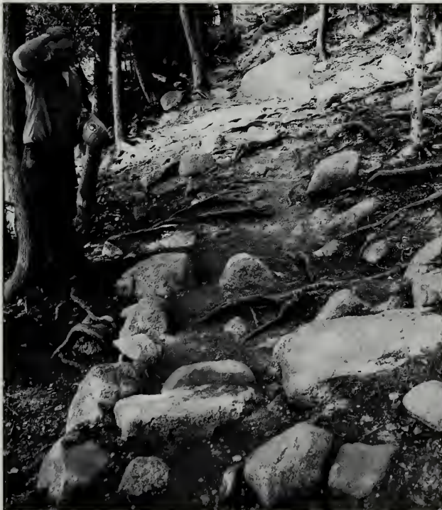
Fig. 39-23 Heavily rooted area and deteriorated tread on the west side of the pond.
