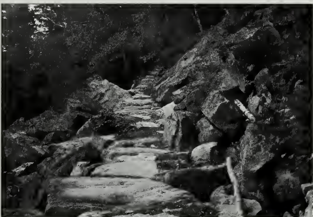
Fig. 3-37 Talus pavement on the Beachcroft Path (#13), circa 1920.
