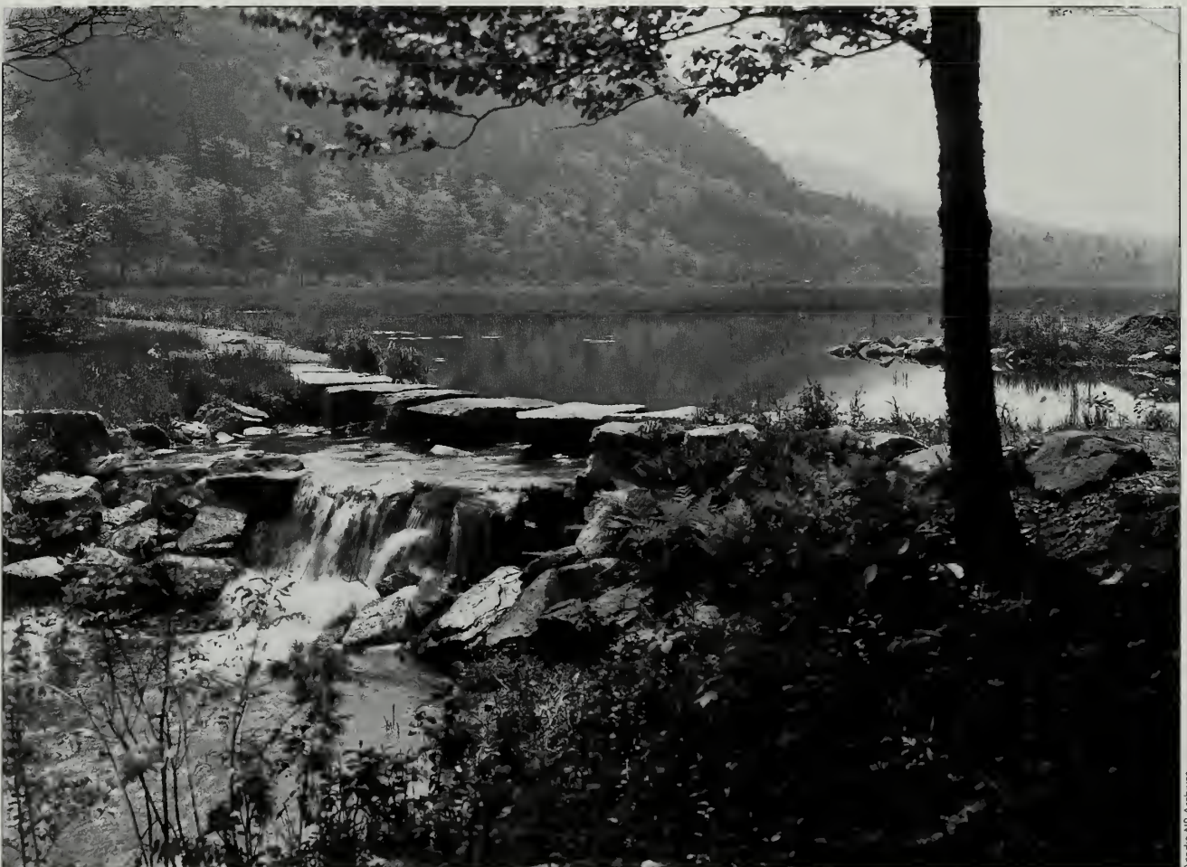
Fig. 5-52 A stream crossing was a typical location for stepping stone use by the early VIA/VIS trail builders. Shown in circa 1916, the stones cross a shallow stream over the dam at the outlet of The Tarn. These stream-style stepping stones proved to be a more durable option than a bridge, as they are still extant nearly ninety years later.
