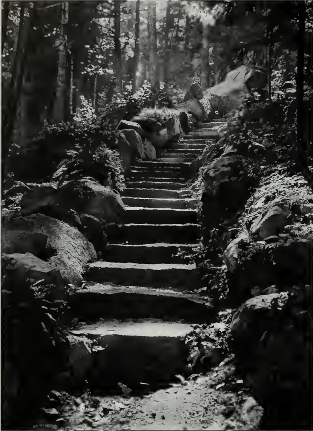
Fig. 7-10 Coping is used with stairs on the Emery Path (#15), circa 1920. There is also an obscure culvert under this staircase.
