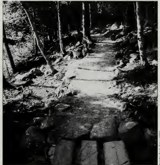
Fig. 39-24 2002 NPS new stone sidewall, gravel, open stone culvert (with temporary wood planks) on west side near section pictured in Fig. 39-23.
