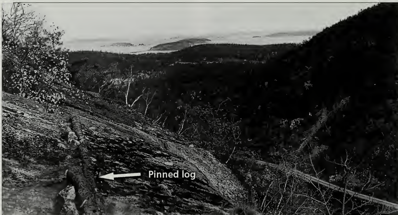
Fig. 8-22 A pinned retaining log on the Ladder Trail (#64) shown in the 1920s.
