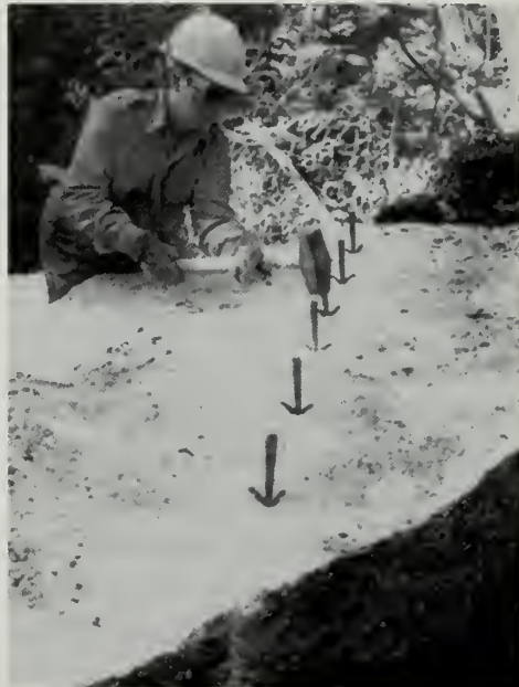
Deb Hofford, SCA-BSP crew of '97 pounds 6 inch wedges to begin splitting a 10-ton slab of granite.
