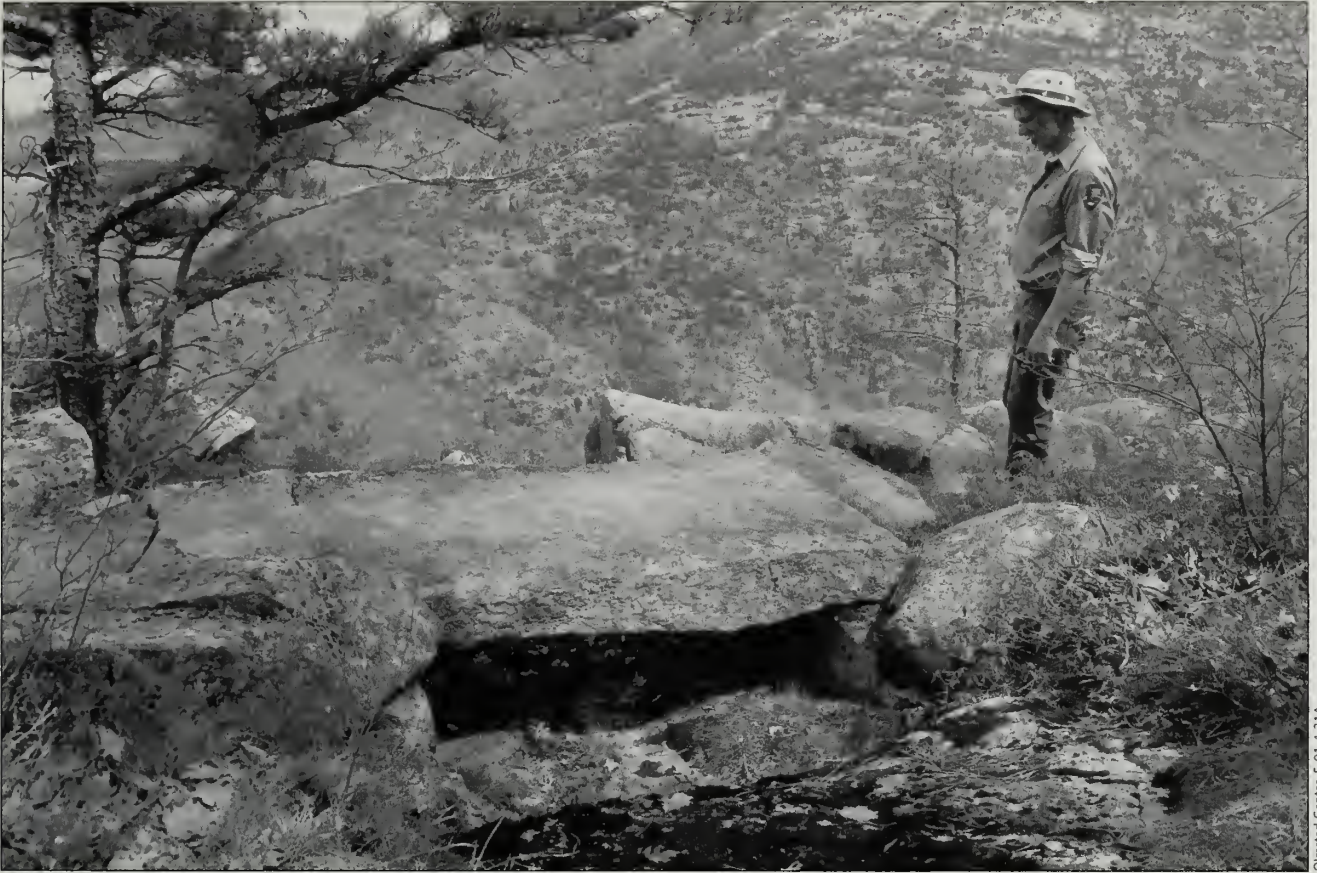
Fig. 4-1 A large capstone culvert on the Schiff Path (#15).
