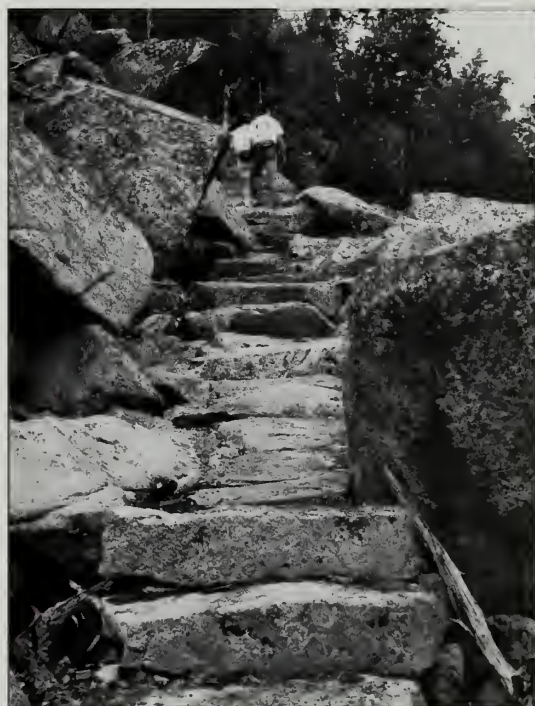
Fig. 349-6 Stone steps and stone pavement through talus slope.
