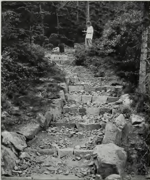
Fig. 6-7 Checks, wall, and rubble in place.
