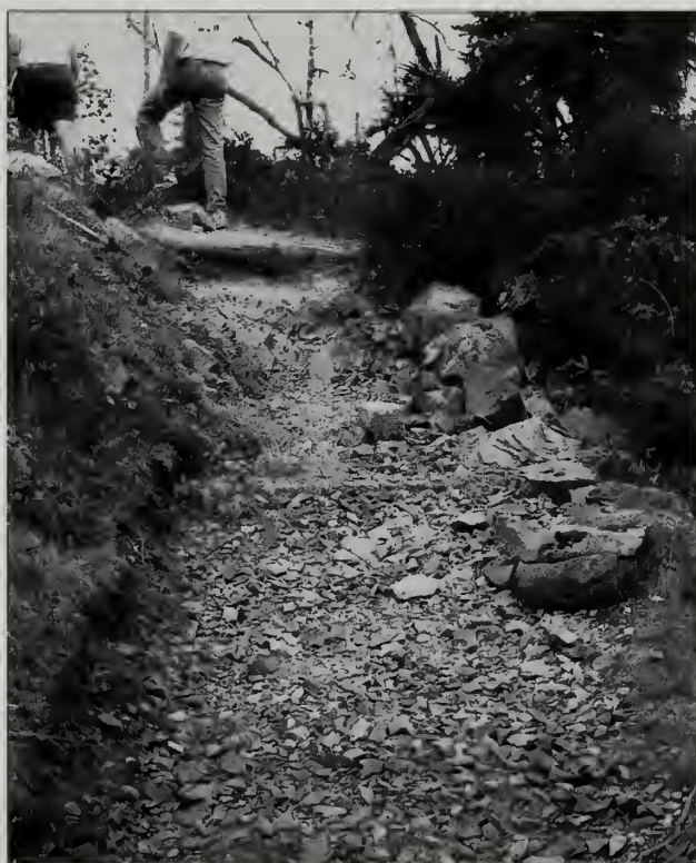
Fig. 6-5 Eroded trail section on the Ocean Path (#3) before check installation.
