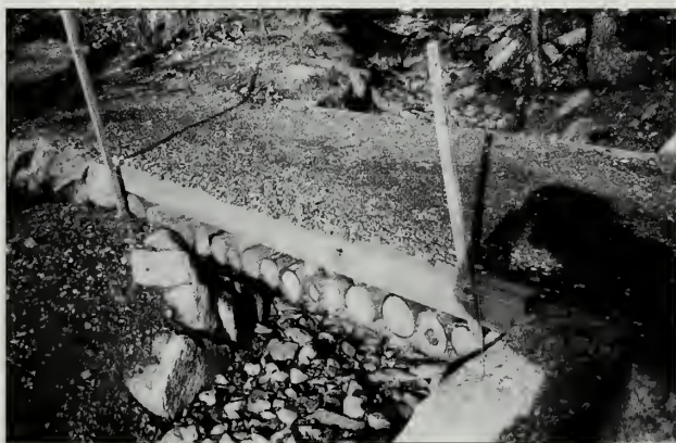
Fig. 5-39 Gravel-surfaced bridge on Jordan Pond Path (#39), constructed in 2001.
