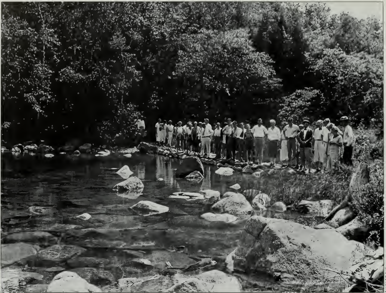
Fig. 3-20 Circa-1934 photograph of a hiking party on Jordan Pond stone causeway that shows the popularity of the area. Refer to Fig. 3-14 for a 1997 view of the causeway after NPS reconstructed and widened it.
