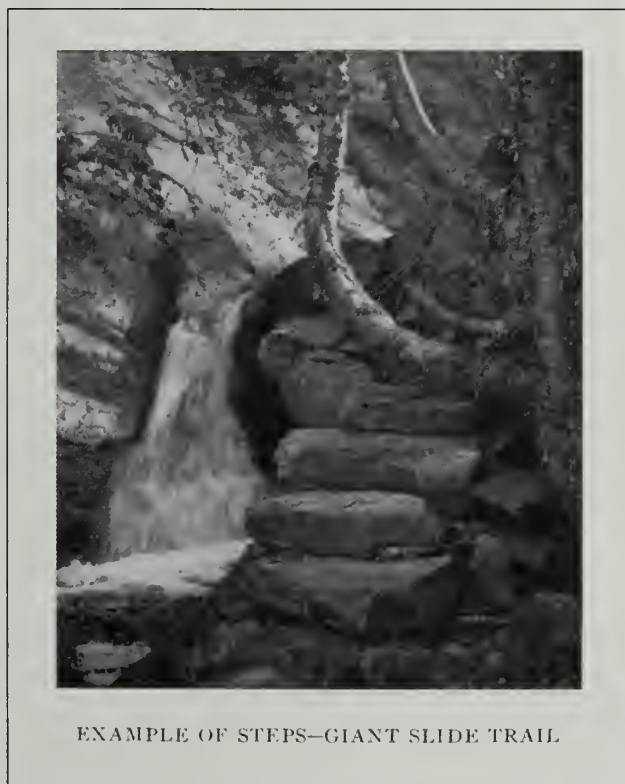
Fig. 6-15 A 1906 image of steps constructed without sidewall or coping stones on the Giant Slide Trail (#63).
