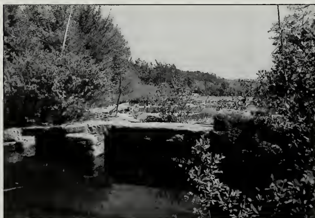
Fig. 5-49 A 1997 view of the Kane & Bridgham Memorial Bridge showing the remaining pieces of the bridge. Rising waters from beaver activity along with ice damage have taken their toll on this structure, and at times it is almost completely submerged.
