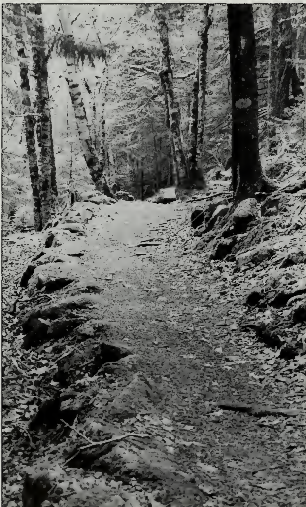
Fig. 3-5 A CCC bench cut with an outside retaining wall on the Valley Trail (#116). Note that the outslope is lost and the tread is wearing.
