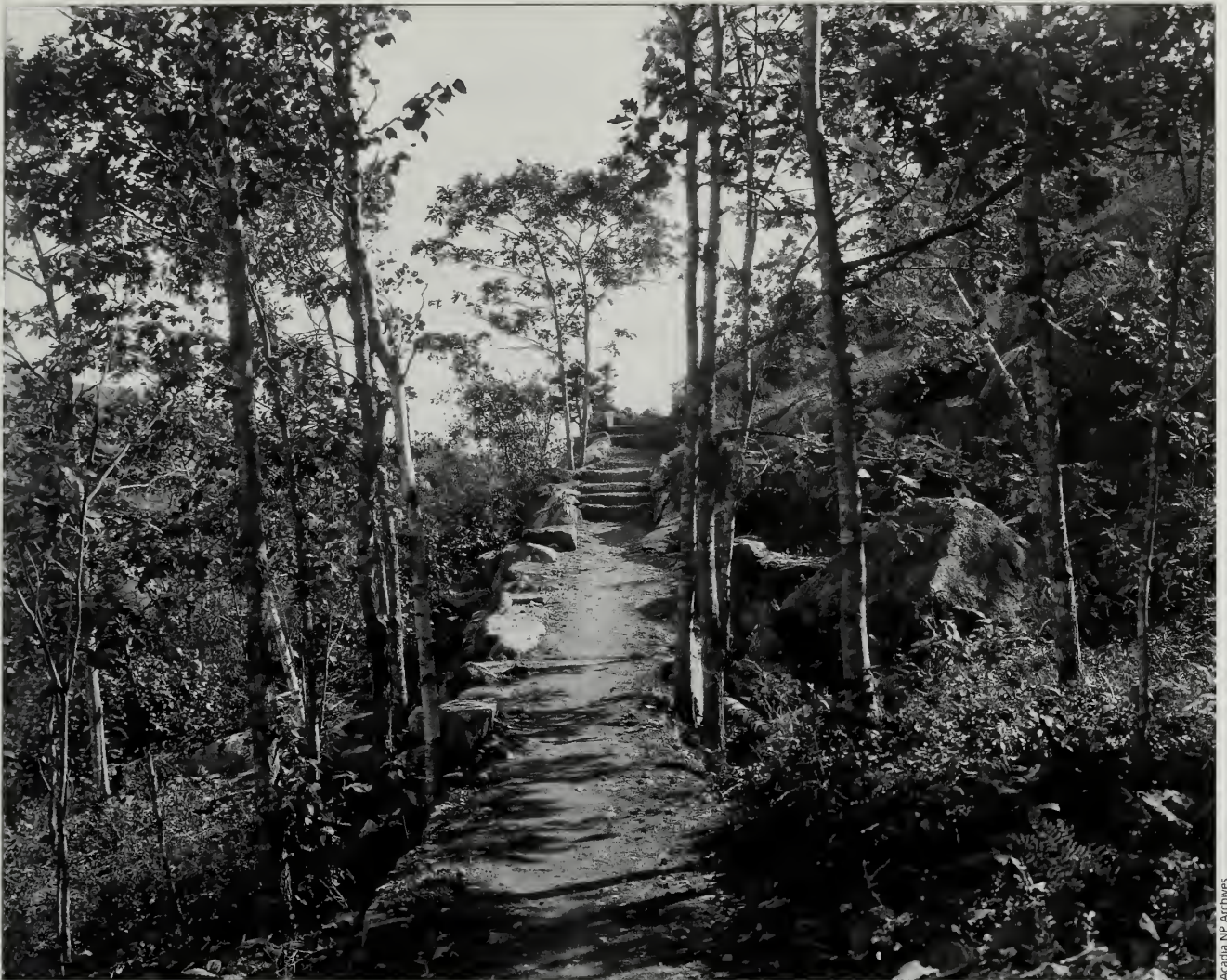
Fig. 6-1 Retaining features on this section of the Schiff Path (#15) include retaining walls and coping stones. These elements hold the tread and steps in place, and provide guidance for the hiker, perhaps preventing a misstep off the trail. Photograph circa 1920.
