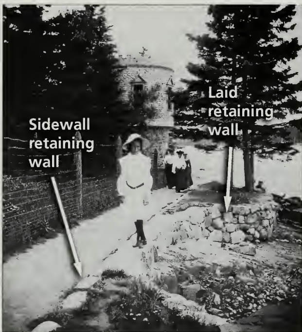
Fig. 6-27 This circa-1890 image of the Shore Path in Bar Harbor (#301) shows the early use of both sidewall and laid retaining walls.
