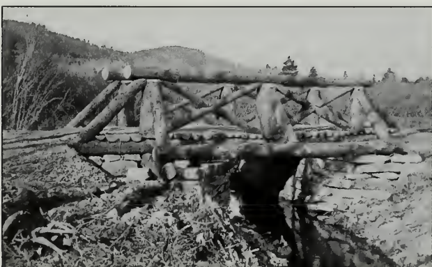
Fig. 5-32 CCC bridge in Great Meadow with stepped-down railings and outrigger bracing, 1930s.
