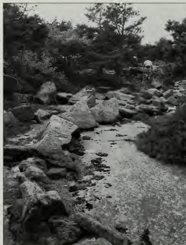
Fig. 6-14 This coping along ledge on the Upper Ladder Trail (#334) was likely constructed by Bar Harbor VIA in the late 1800s.
