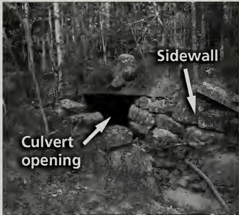
Fig. 4-12 A VIA/VIS or CCC graveled-over road culvert near the Jesup Path (#14) between The Tarn and Sieur de Monts Spring.
