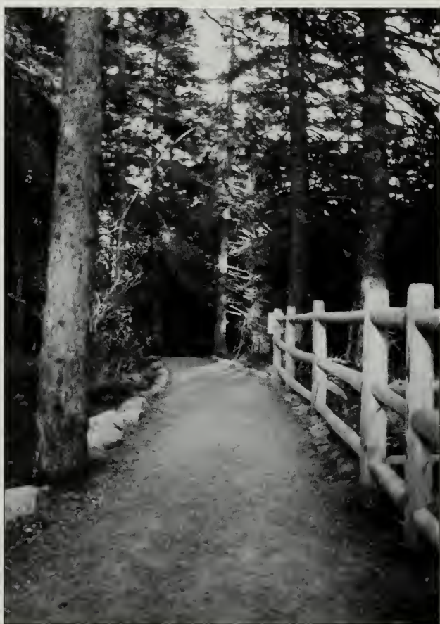
Fig. 3-31 New gravel tread was installed by the NPS on the rehabilitated Bass Harbor Head Light Trail (#129) in 1997.
