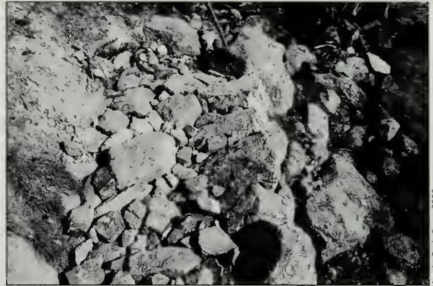
Fig. 6-43 Stone retaining wall construction on Jordan Pond Path (#39). The top course of stones are sloped in and set header-style with high contact, and the core is properly blocked.
