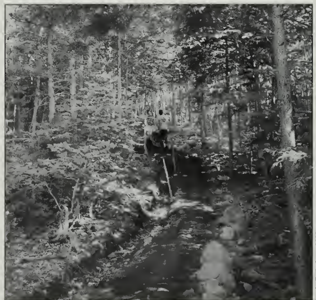
Fig. 4-35 Ditch and fill on Deer Brook Trail (#51) with tread constructed of material taken from the ditch. Sides of the ditch are sloped and the ditch (in foreground) has been angled properly.
