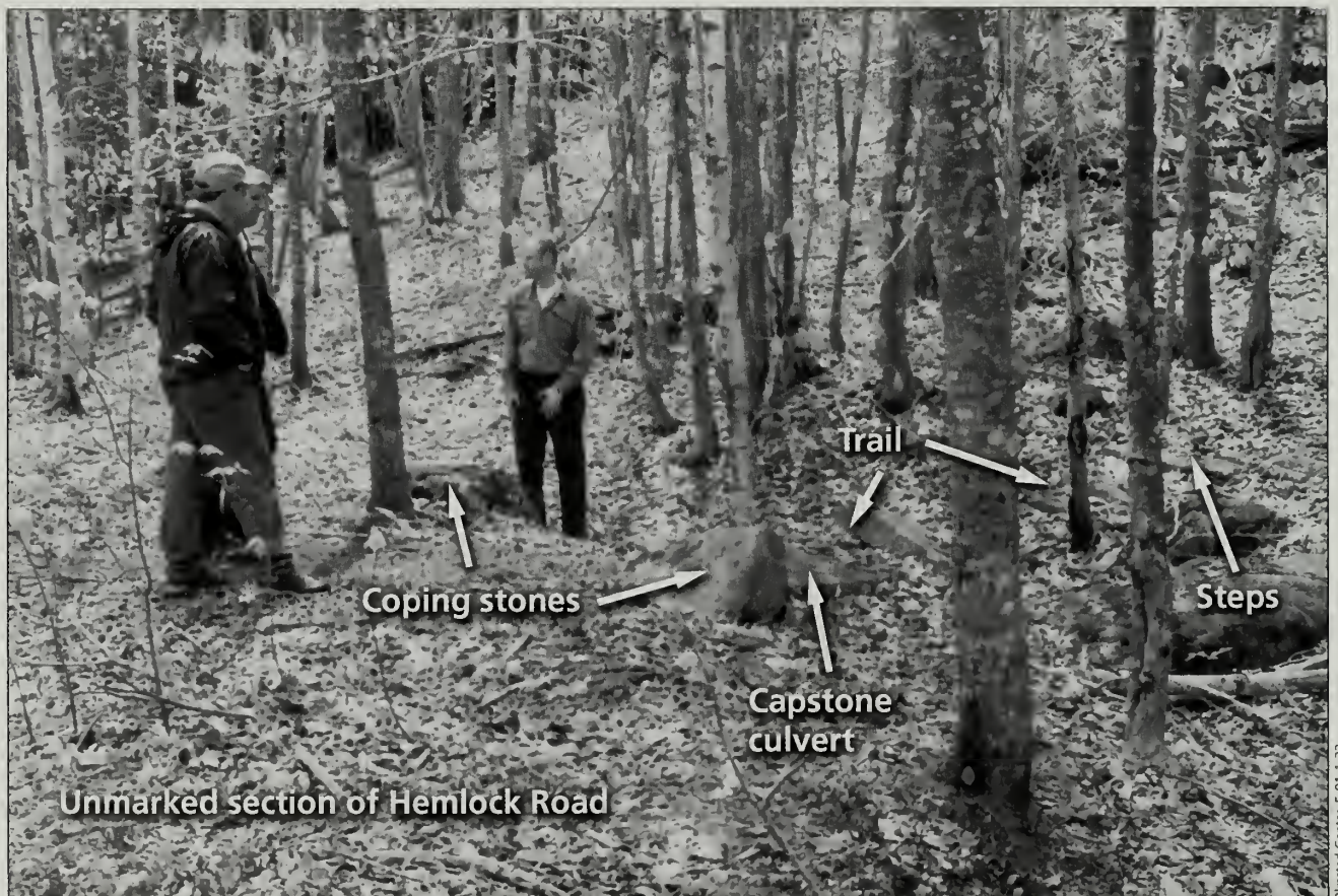
Fig. 349-3 The entrance to the Homans Path is on an unmarked section of Hemlock Road (#377), marked by two large coping stones. Constructed VIA sonework is prevalent along the trail, and the first features at the trailhead include a capstone culvert over the road's drainage ditch, and followed by a series of steps.
