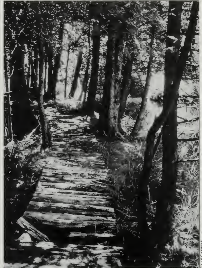
Fig. 5-3 This bogwalk on the Upper Hadlock Pond Trail (#501), shown here in 1967, was likely built by the Northeast Harbor VIS in the 1930s or 1940s. This bogwalk is more similar to a bridge, with its stringers and corduroy decking, than it is to the contemporary style of bogwalk used in Acadia.
