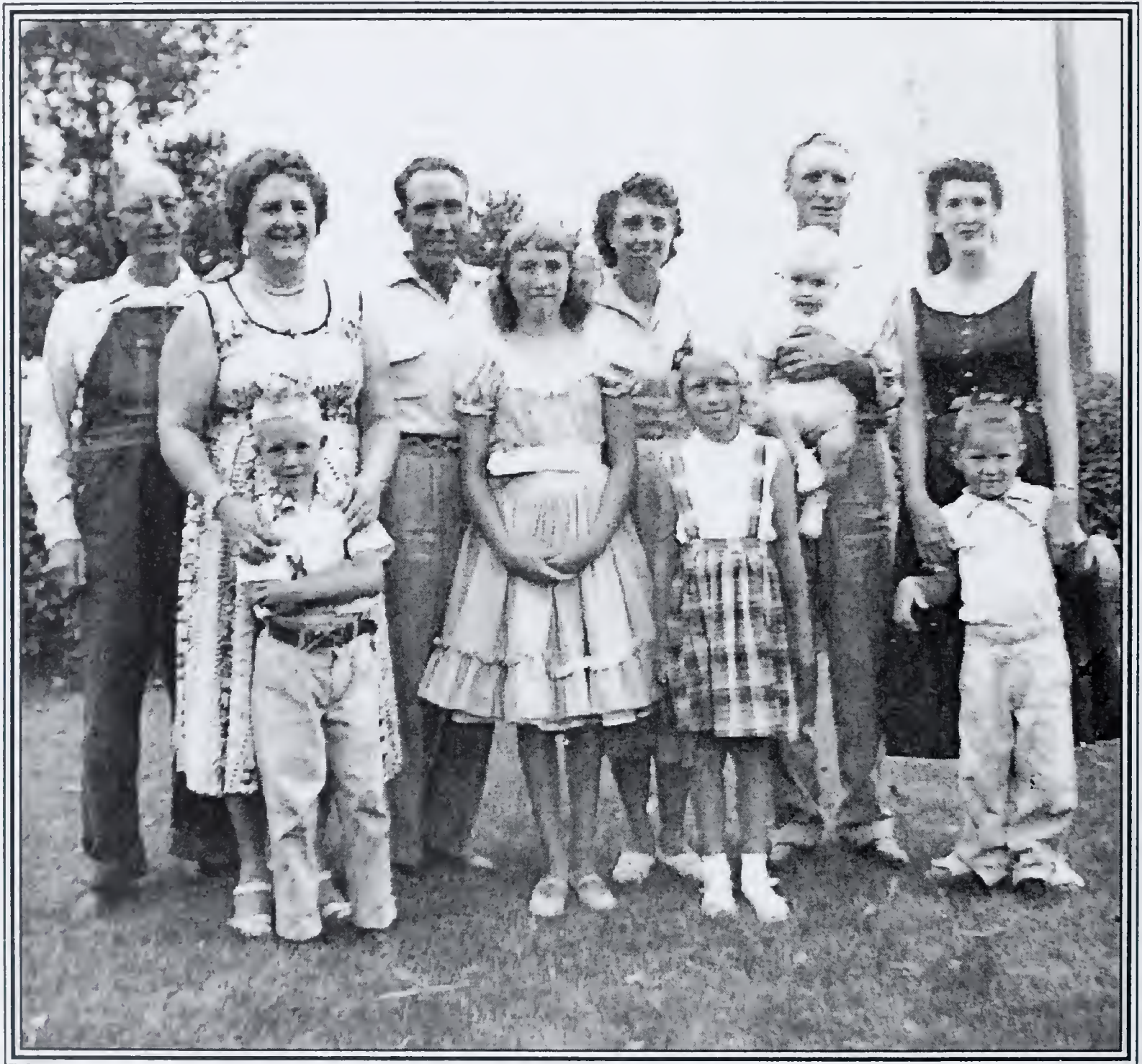
1955 Art Hawkes' family at the Idaho Falls Power Plant.
