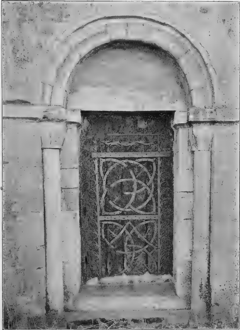
LITTLE HORMEAD CHURCH : BLOCKED NORTH DOORWAY
