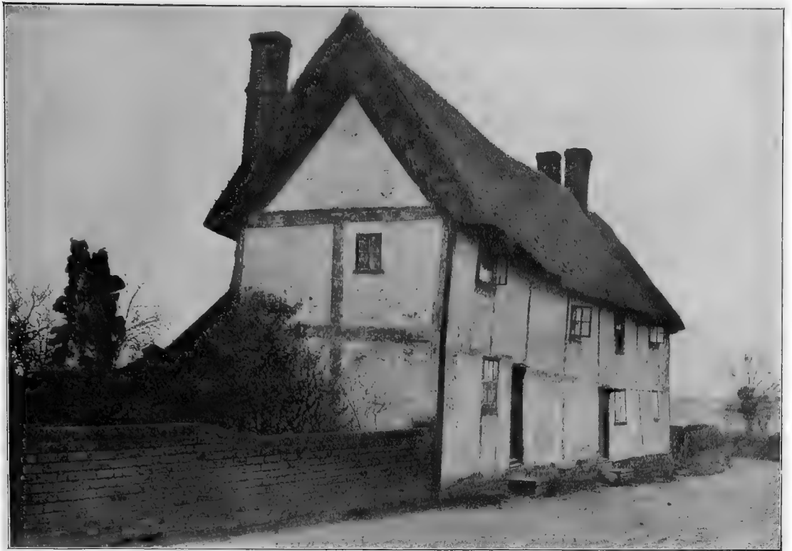
ALBURY · HALF-TIMBERED HOUSE ADJOINING THE CHURCHYARD
