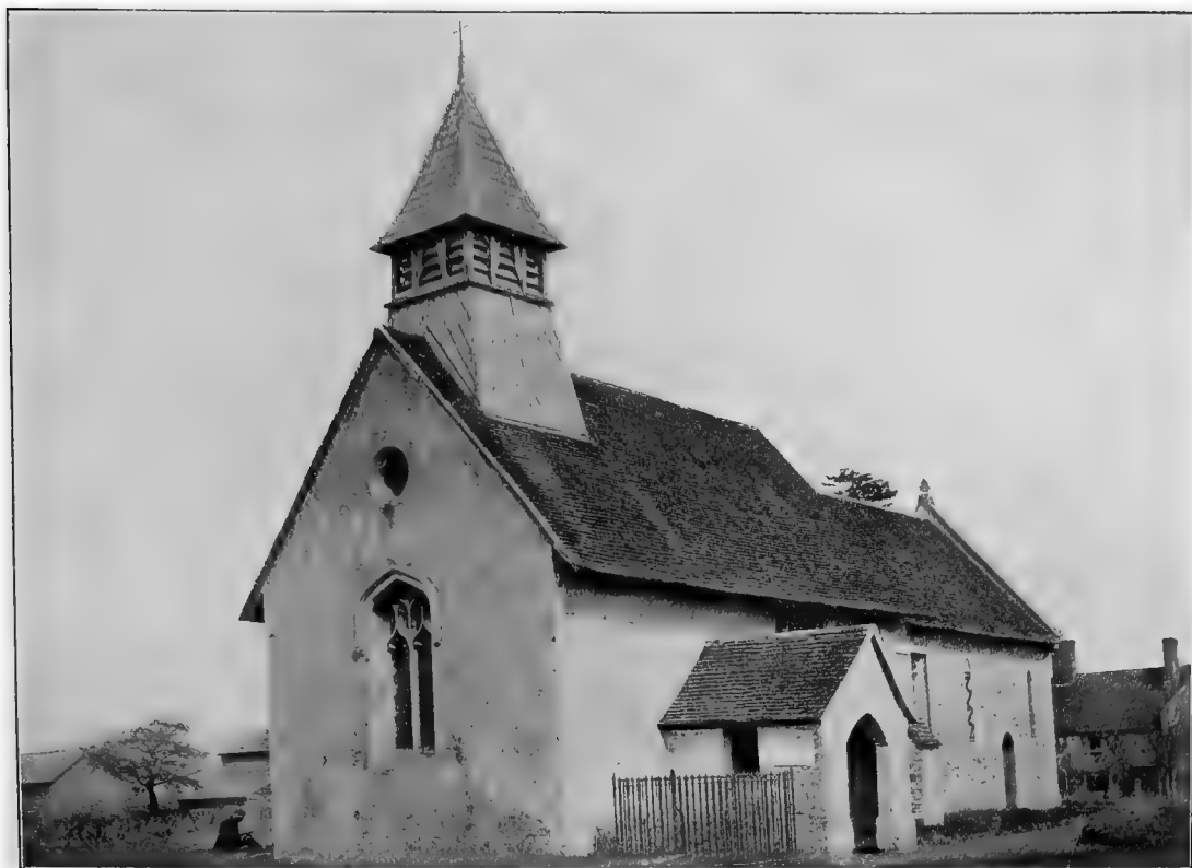
LITTLE HORMEAD CHURCH FROM THE SOUTH-WEST
