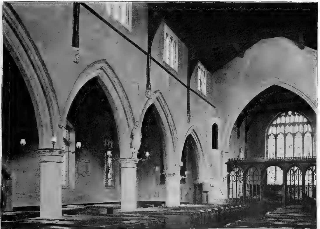
MUCH HADHAM CHURCH : THE NORTH ARCADE
